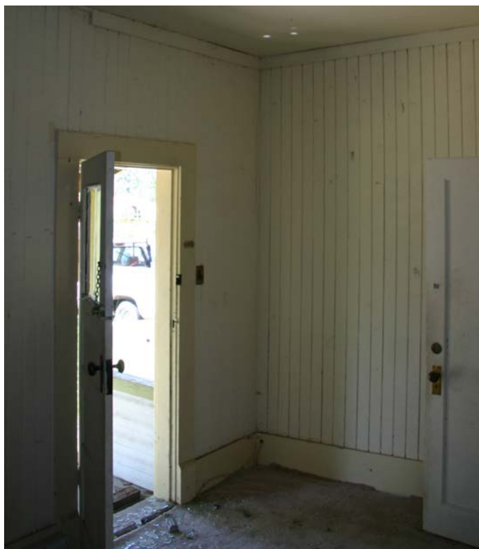
Surviving original v-joint panelling on walls and ceiling of front hall, showing original main entrance door to the left.
