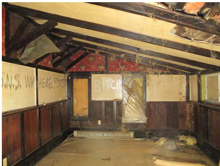
Interior space of the dining room (east early addition) showing exposed shed roof rafters with angle web wood members.
