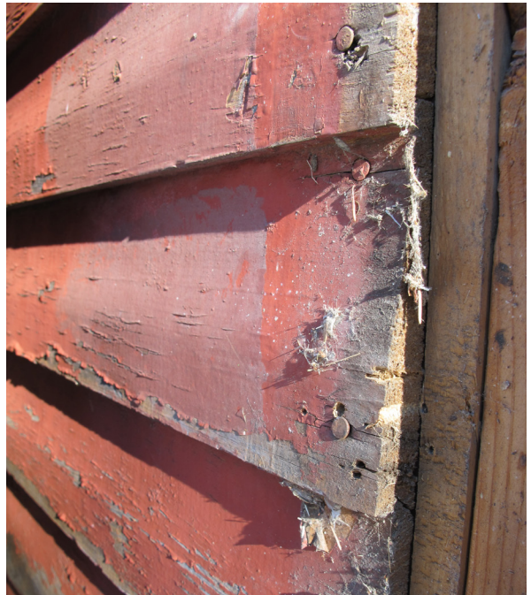
Photos showing typical deteriorated condition of exterior wall cladding, as well as roof soffit and corner board trims.
