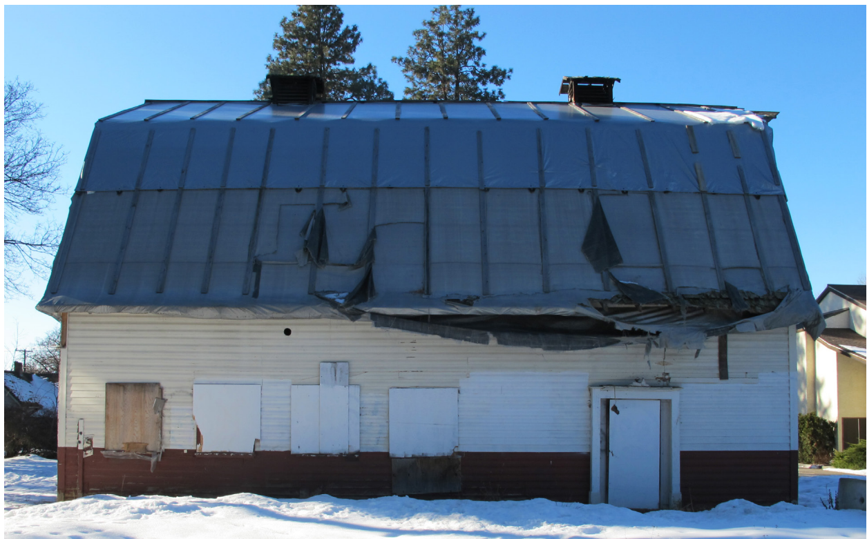
Archival photo showing east elevation of the Surtees Barn (top), with small log house in the background (demolished). Photo showing existing condition of east elevation of the Surtees Barn (bottom); note in the background showing a portion of the Surtees House to the left, and the St. Andrew's Church to the right.
