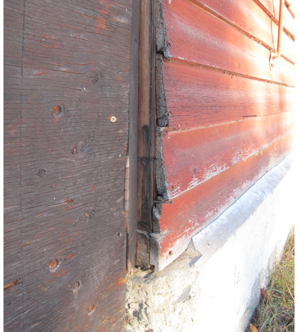
Photos showing typical deteriorated condition of exterior wall cladding above concrete foundation walls. Note profile of original drop siding (top right).
