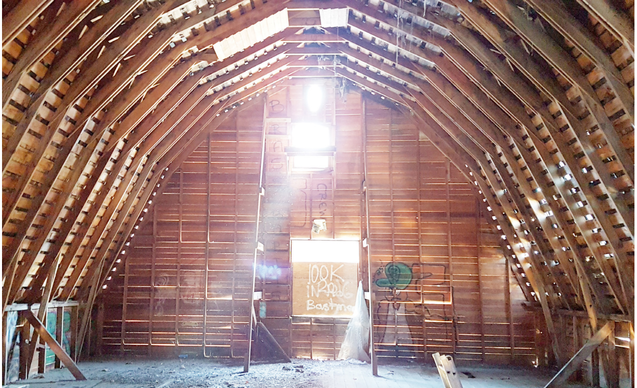
Photos showing exposed gambrel roof structure of the Surtees Barn.
