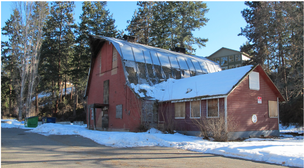
Photos showing north elevation of Surtees Barn, as viewed from northeast (top) and northwest (bottom). Note hill with mature landscape in the background.
