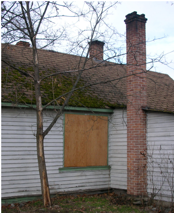
Southwest corner view of the house showing later addition, with exterior brick chimney in the foreground, and two original interior chimney stacks in the background.
