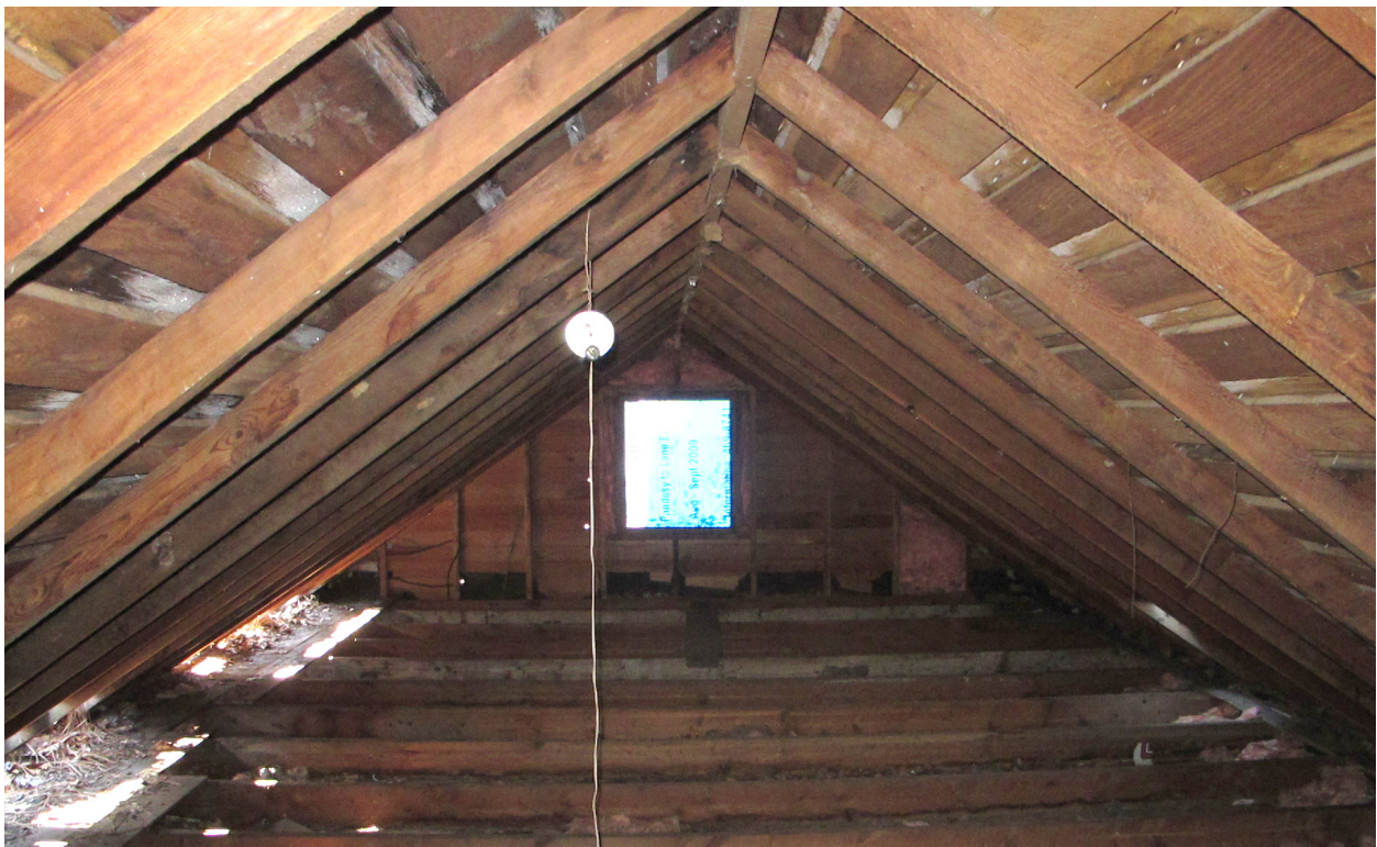
Photos showing side-gabled roof structure of the Surtees Barn extension, from exterior (top) and interior (bottom) side.
