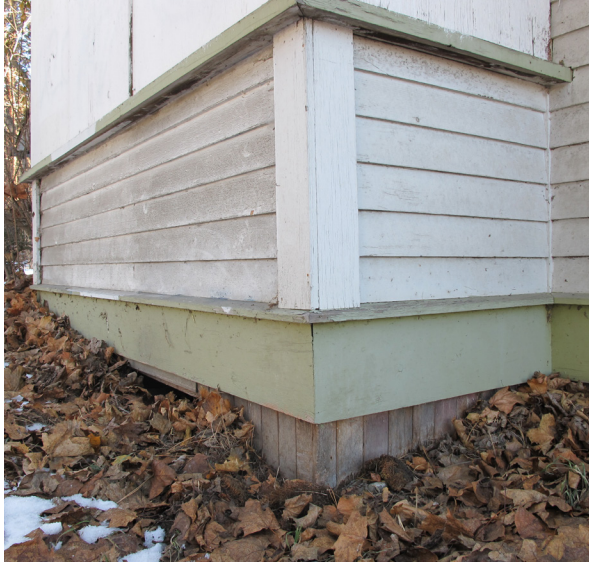
Lower portion of bay window at north elevation, showing wood lapped siding, window sill, and board trims. Note that foundation wall is clad in later vertical siding.
