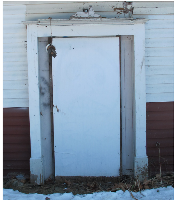
Photos showing original, existing door assembly at west return of south elevation (top), and later door surround trim at east elevation (bottom).
