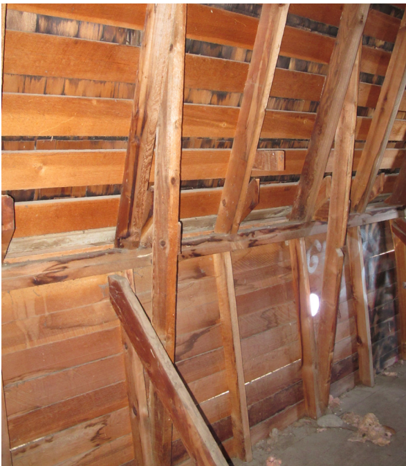
Interior side of the wall-to-roof interface, showing typical existing condition of the original wood materials.
