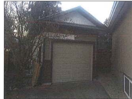
3 A1 CLOSE UP OF EXISTING GARAGE
