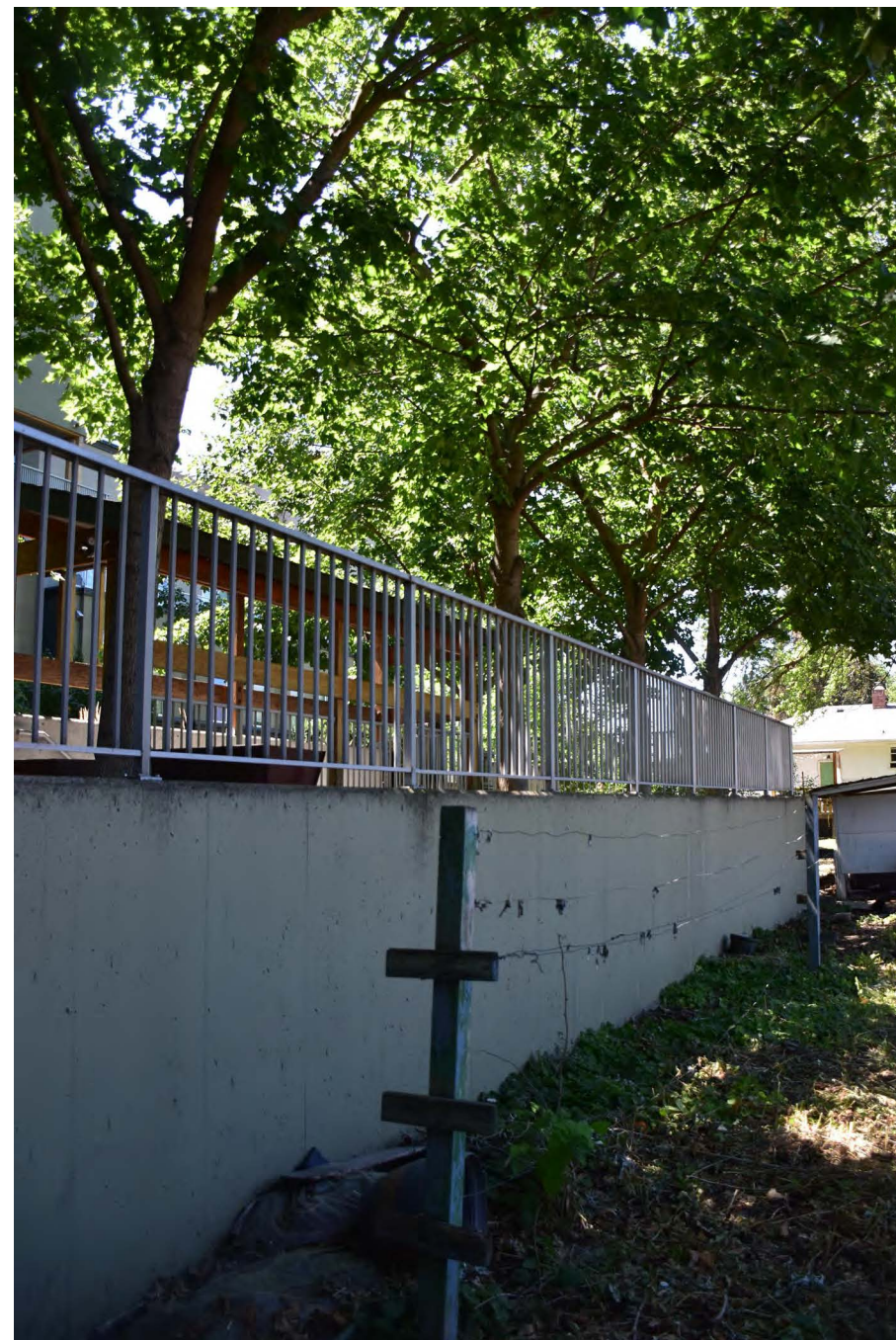
SOUTH YARD - RETAINING WALL - 1.8M HIGH
