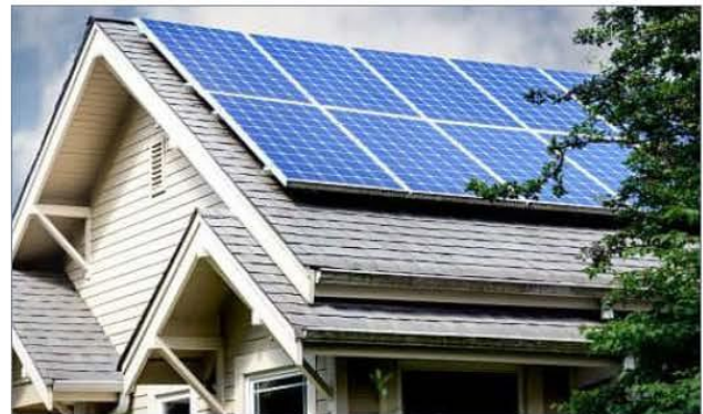
Figure 25: Place solar panel installations on property elevations, roof planes, or ground locations that respect the landscape and minimize visibility from the street.
