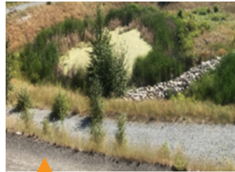
Stormwater ponds are constructed to capture water, reduce downstream peak flows and improve the quality of water entering the creek or water body.
