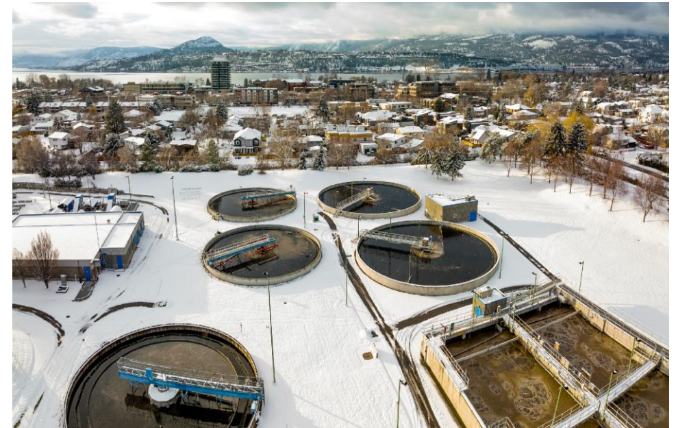
Secondary Clarifiers Raymer Wastewater Treatment Plant
