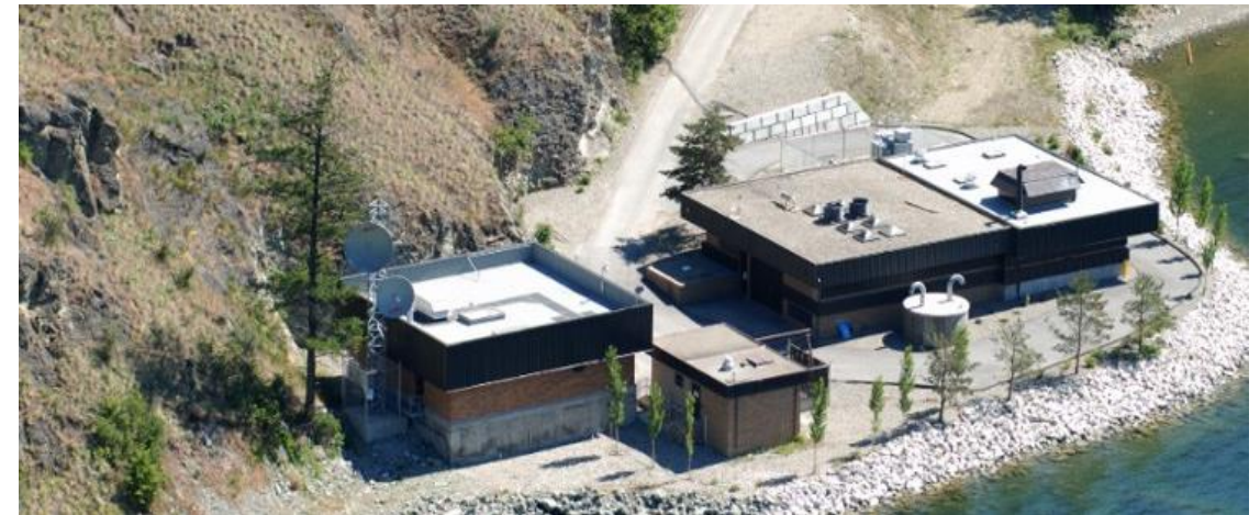
Poplar Point Lake Intake & Pump Station
