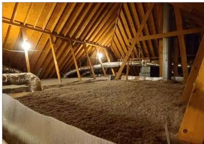
Figure 24: Enhance insulation, particularly in attic and basement spaces.
