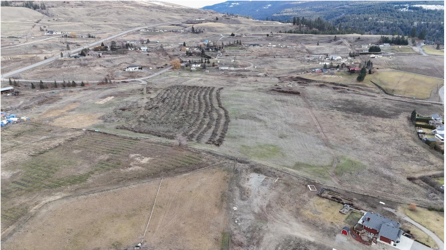
Photo #1: December 2023 aerial image of soil and fill placed and ready to be spread from North (left) to South (right).
