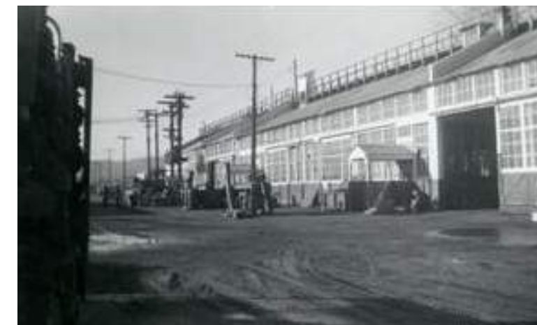
Figure 63. Looking south. The Machine Shop, 1940s. From the Simpson Family Fonds
