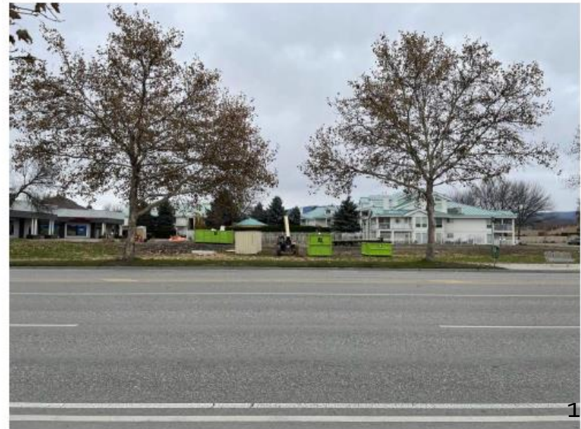
D EXIST. VIEW FROM GORDON, LOOKING NORTH EAST
