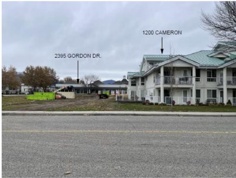
A EXIST. VIEW FROM CAMERON, LOOKING NORTH
