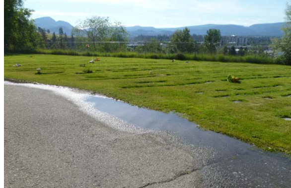
Figure 37: Ponding of water due to a break in an irrigation line by the Bennett Memorial.
