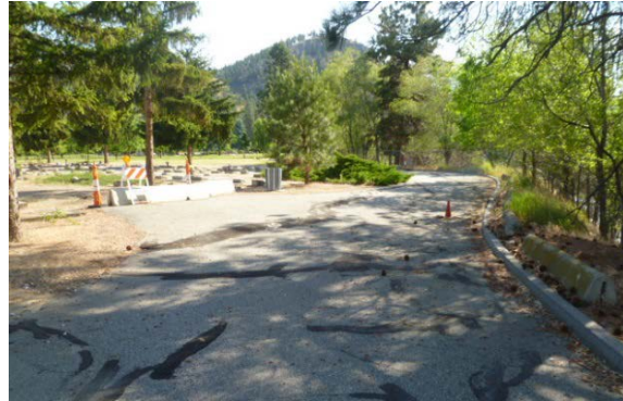
Figure 31: Ground movement has buckled the road forming the southern boundary of KMPC.
