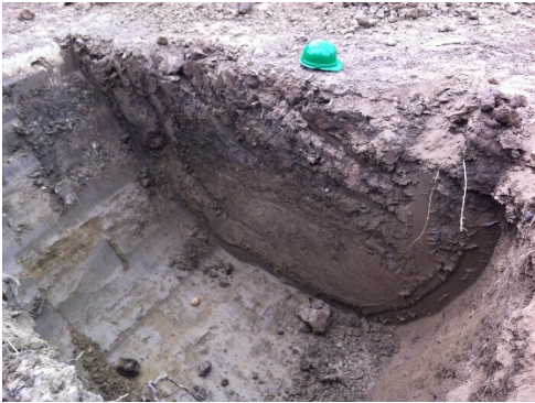
Figure 84: Example photo of test grave to determine suitability of the ground
