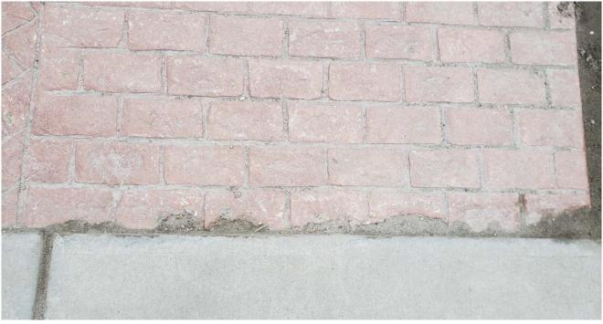
Figure 15: Cracking of stamped concrete paving along edge of municipal sidewalk at Southeast corner of garden, off Clement Avenue
