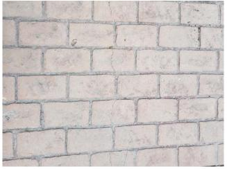
Figure 27: Small crack in surface of stamped concrete paving
