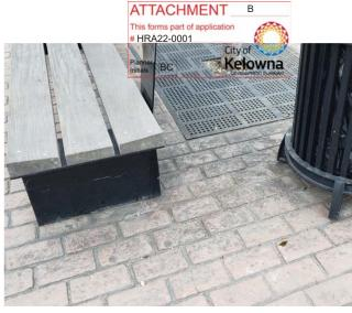
Figure 26: Darkening on stamped concrete paving
