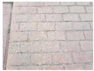
Figure 28: Salt damage along East side of plaza
