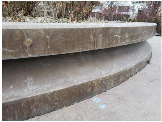
Figure 11: Cracking and scratches along top edge of raised planter
