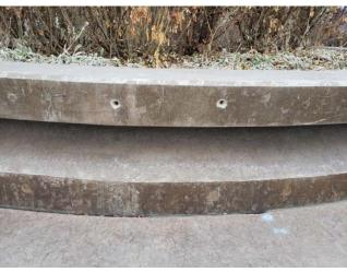
Figure 12: Holes in wall of raised planter
