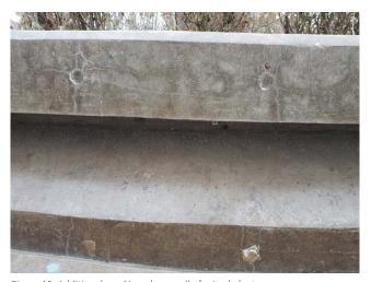
Figure 13: Additional cracking along wall of raised planter
