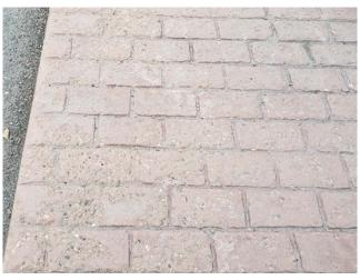
Figure 17: Salt damage along East pathway bordering asphalt parking area
