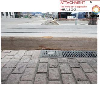
Figure 21: Chip damage on front of timber bench slat
