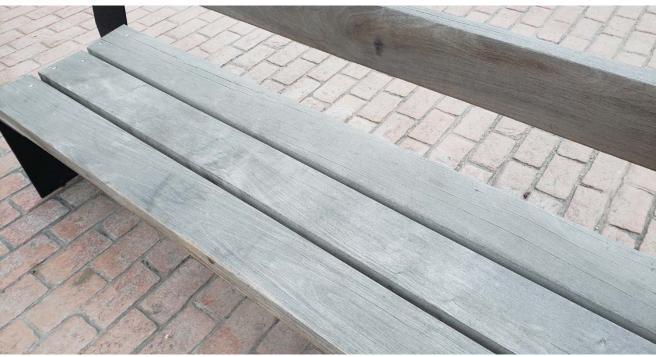
Figure 22: Timber checking on rear bench slat
