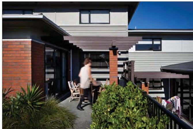
Figure 22: Rooftop patios provide a unique private outdoor space, and should include parapets with railings (3.1.4 f).
