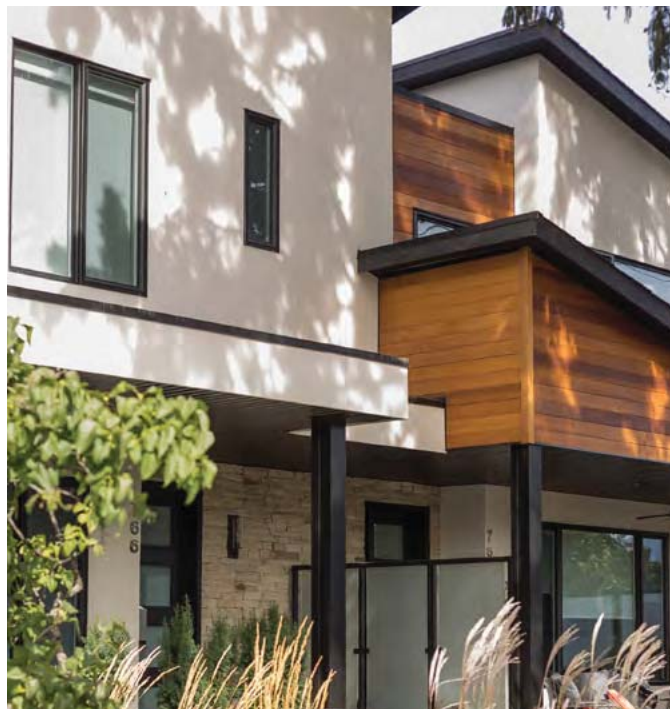
Figure 30: Break down the massing of large buildings through articulation of individual units and avoid symmetry (3.3.2 a).
