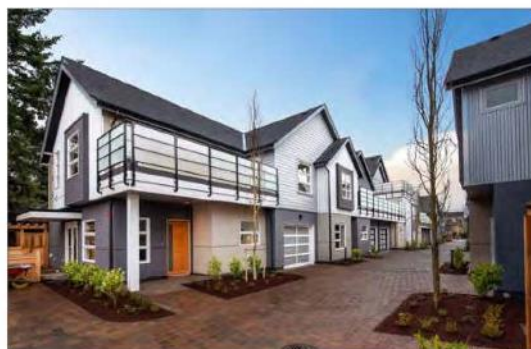
Figure 23: Example of internal roadway designed with high quality pavement materials and strategic landscaping placement (3.1.5 a).
