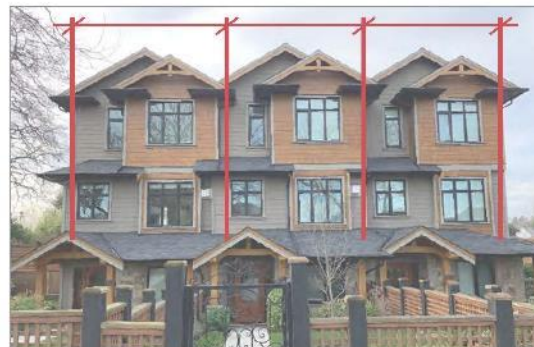
Figure 26: Example of facades and entrance features designed to articulate individual units (3.2.6 a).
