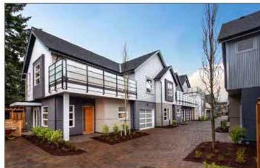
Figure 23: Example of internal roadway designed with high quality pavement materials and strategic landscaping placement (3.1.5.a).
