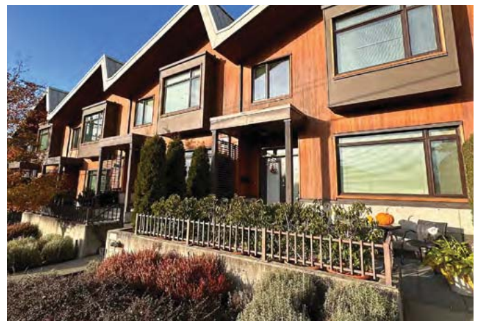
Figure 34: Have landscaped areas to soften the interface with the street and open spaces (3.3.3 e).
