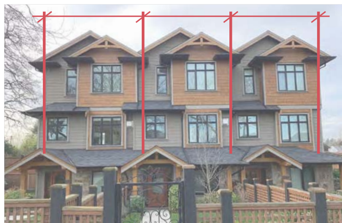
Figure 26: Example of facades and entrance features designed to articulate individual units (3.1.6 a).
