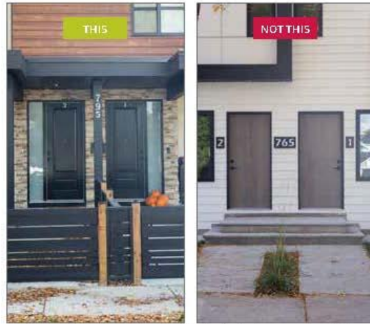
Figure 37: Design facades to articulate individual units using entrance features, roofline features, and other architectural elements (3.3.6 a).
