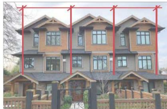
Figure 26: Example of facades and entrance features designed to articulate individual units (3.1.6 a).
