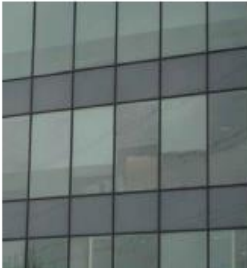
TYPICAL SPANDREL GLASS: LIGHT GREY REFLECTIVE
