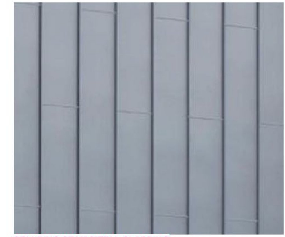
STANDING SEAM METAL CLADDING
