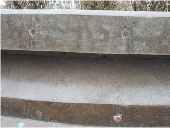
Figure 13: Additional cracking along wall of raised planter
