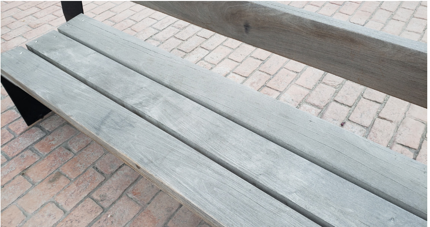
Figure 22: Timber checking on rear bench slat
