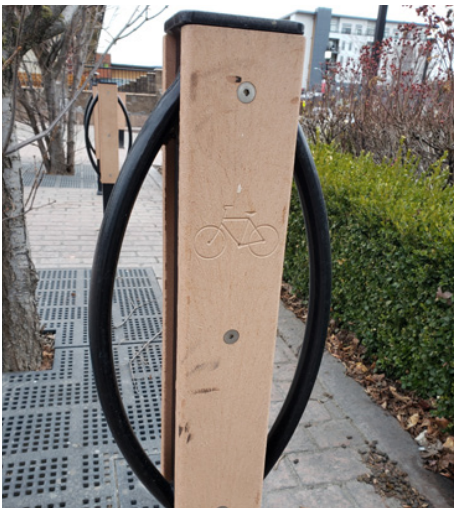
Figure 23: Scuffing and wear on bike rack posts
