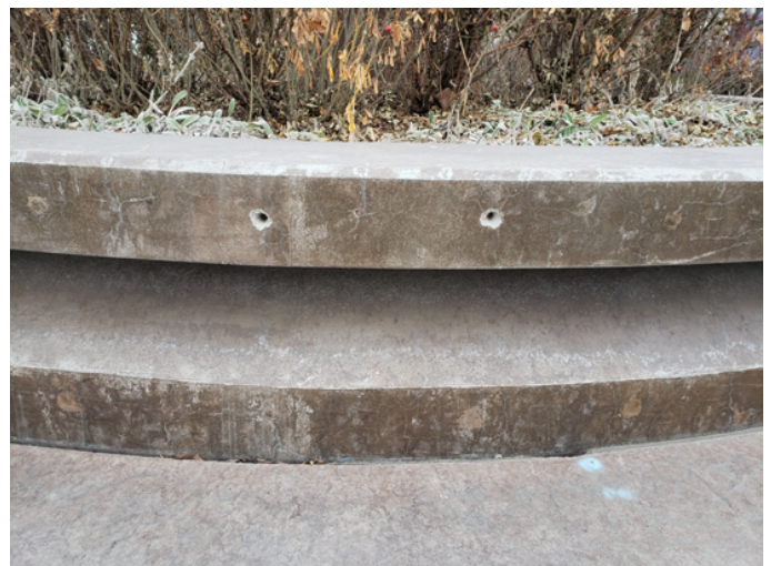
Figure 12: Holes in wall of raised planter
