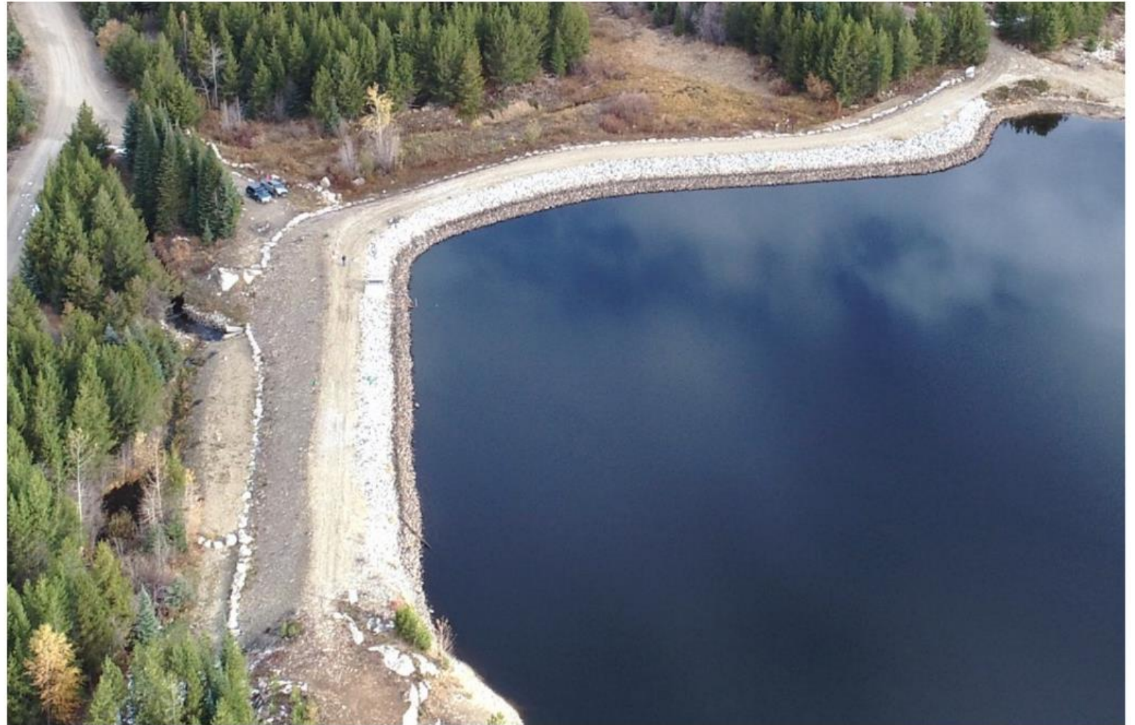
Figure 2-9: Turtle Lake North Outlet Dam – Oblique photograph of dam (October 2021)
