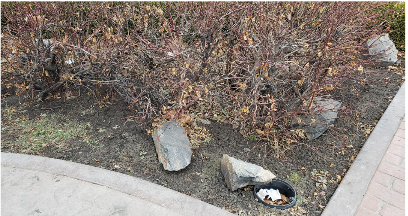
Figure 10: Irrigation valve box missing lid and garbage behind roses in North planting bed. Another valve box was missing a lid in the southwest planting bed.
