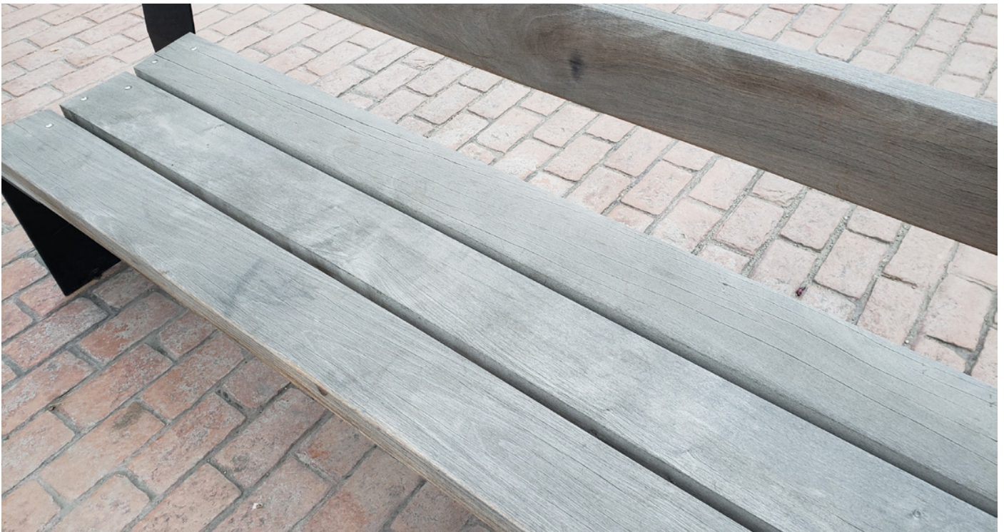
Figure 22: Timber checking on rear bench slat
