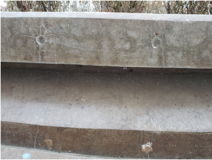
Figure 13: Additional cracking along wall of raised planter
