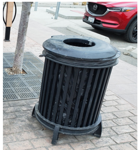
Figure 24: Chipping of powdercoat along rim of waste receptacle
