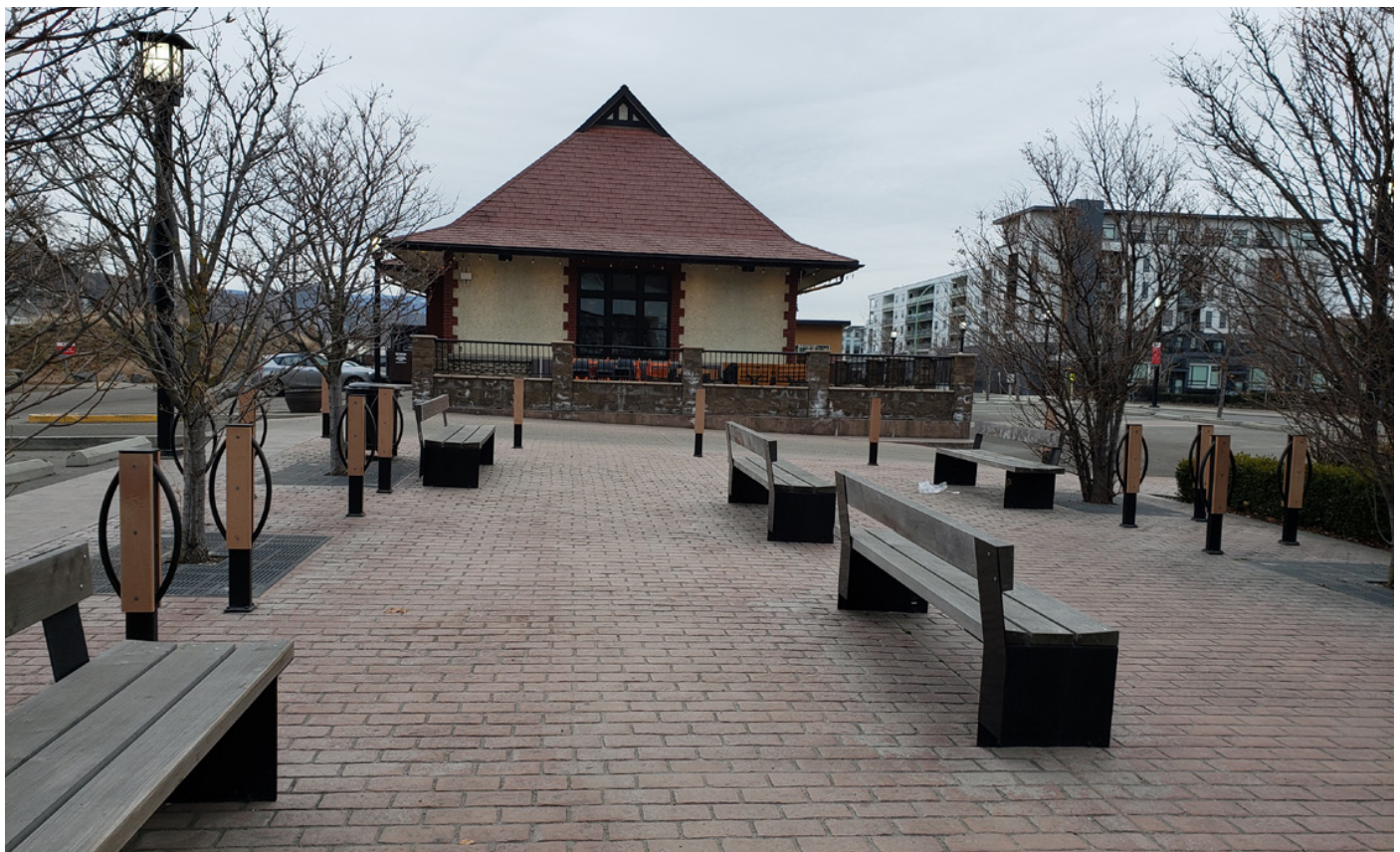
Figure 19: View of the plaza area from Ellis Street
