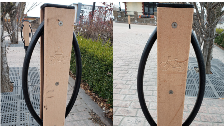
Figure 23: Scuffing and wear on bike rack posts
