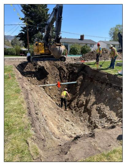
Figure 2: Photo of excavated service trench in Central Rutland Sewer Connection Area.
