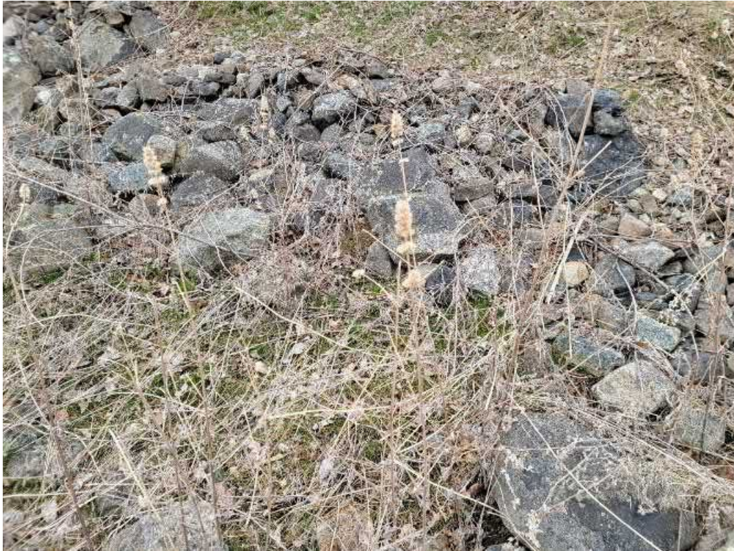
Photo 1.15: Fractured rock within the south limits of the fill placement area
