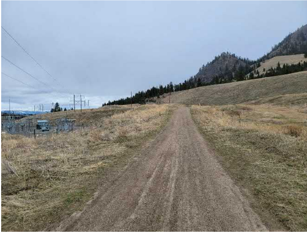
Photo 1.3: Access road and FortisBC electrical substation and transmission line
