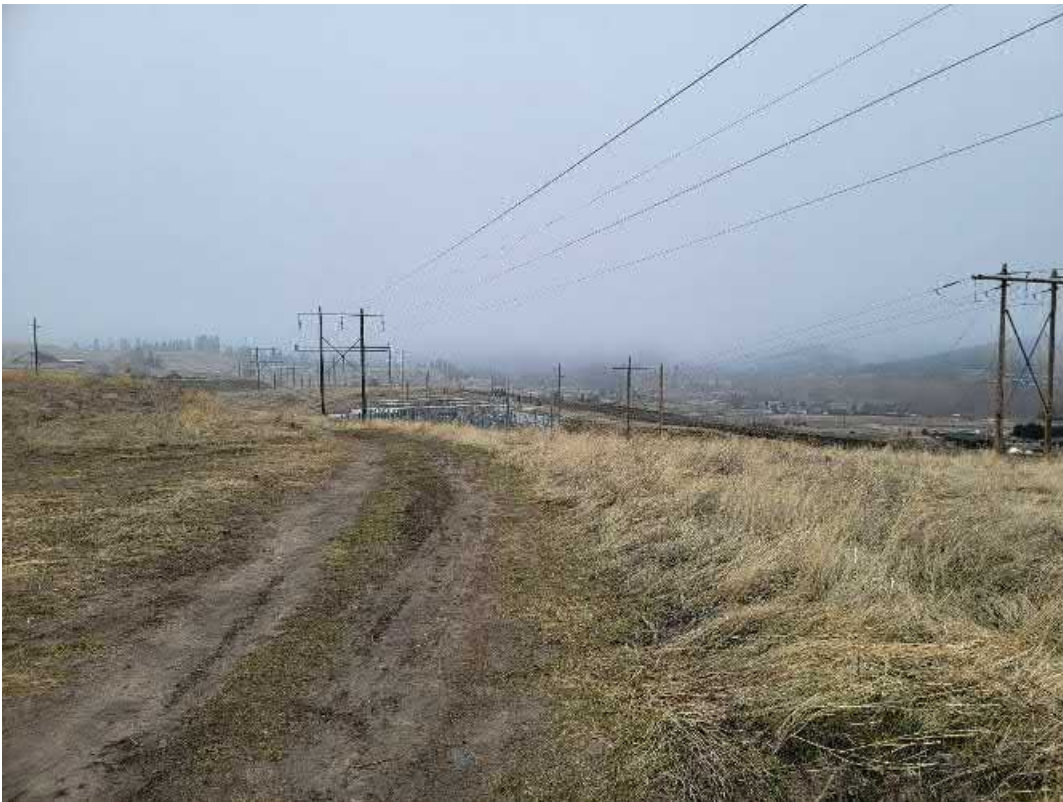
Photo 1.24: Site access and overhead electrical transmission lines west of the fill placement area
