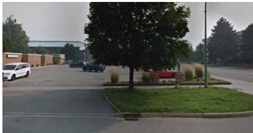
4 VIEW OF CORNER FROM LAWRENCE AVE
