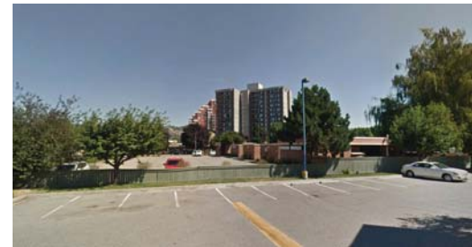
8 VIEW FROM ADJACENT PARKING LOT
