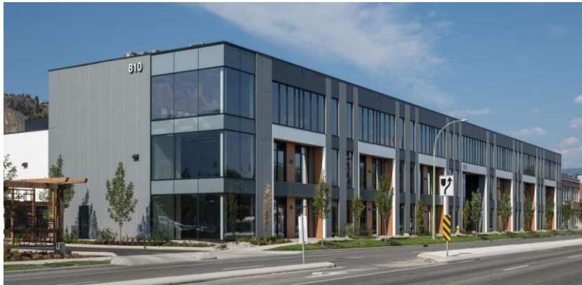
IntraUrban Powerhouse – Industrial (Summer 2021)
