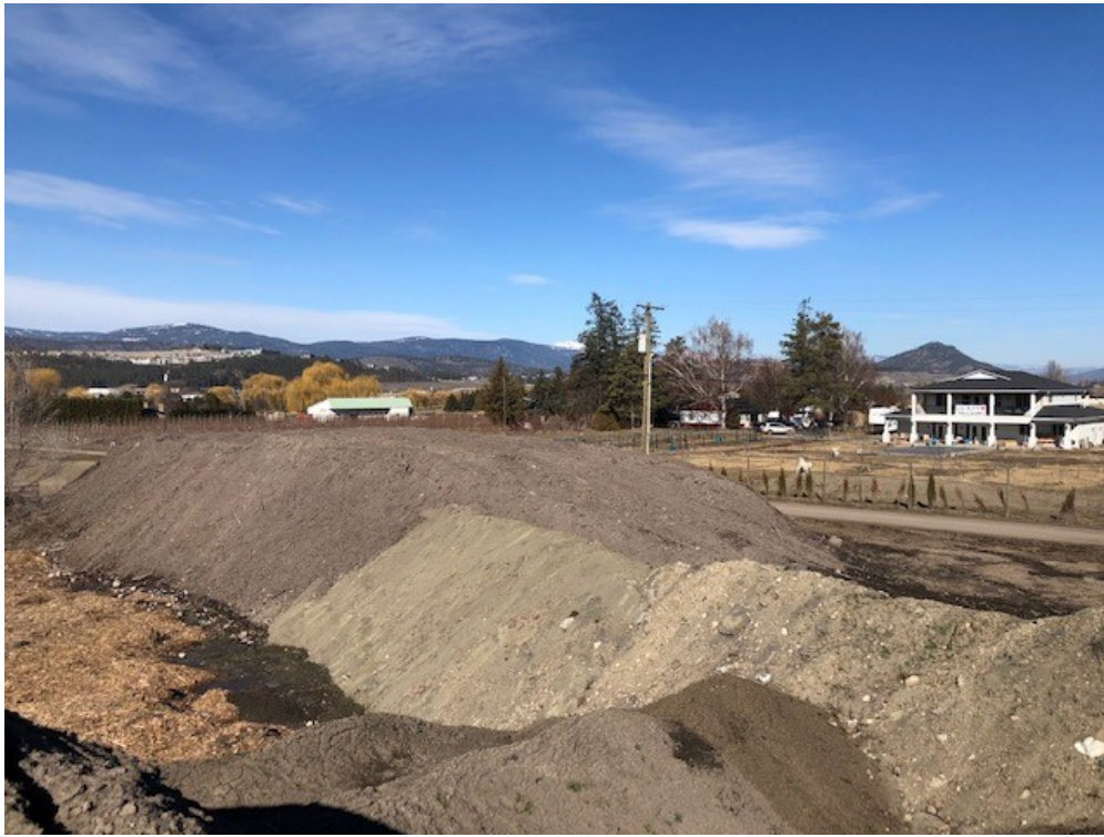
Photo 6. Berm constructed to reduce noise pollution
