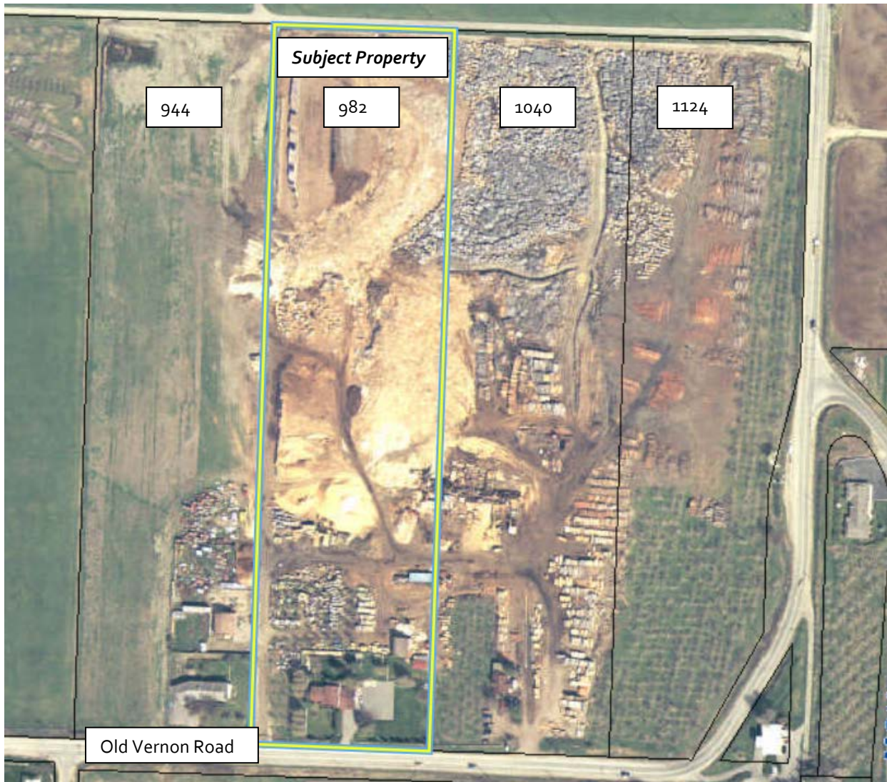
Air Photo 7 – Air photo 2000 of subject property and neighbouring lots.
