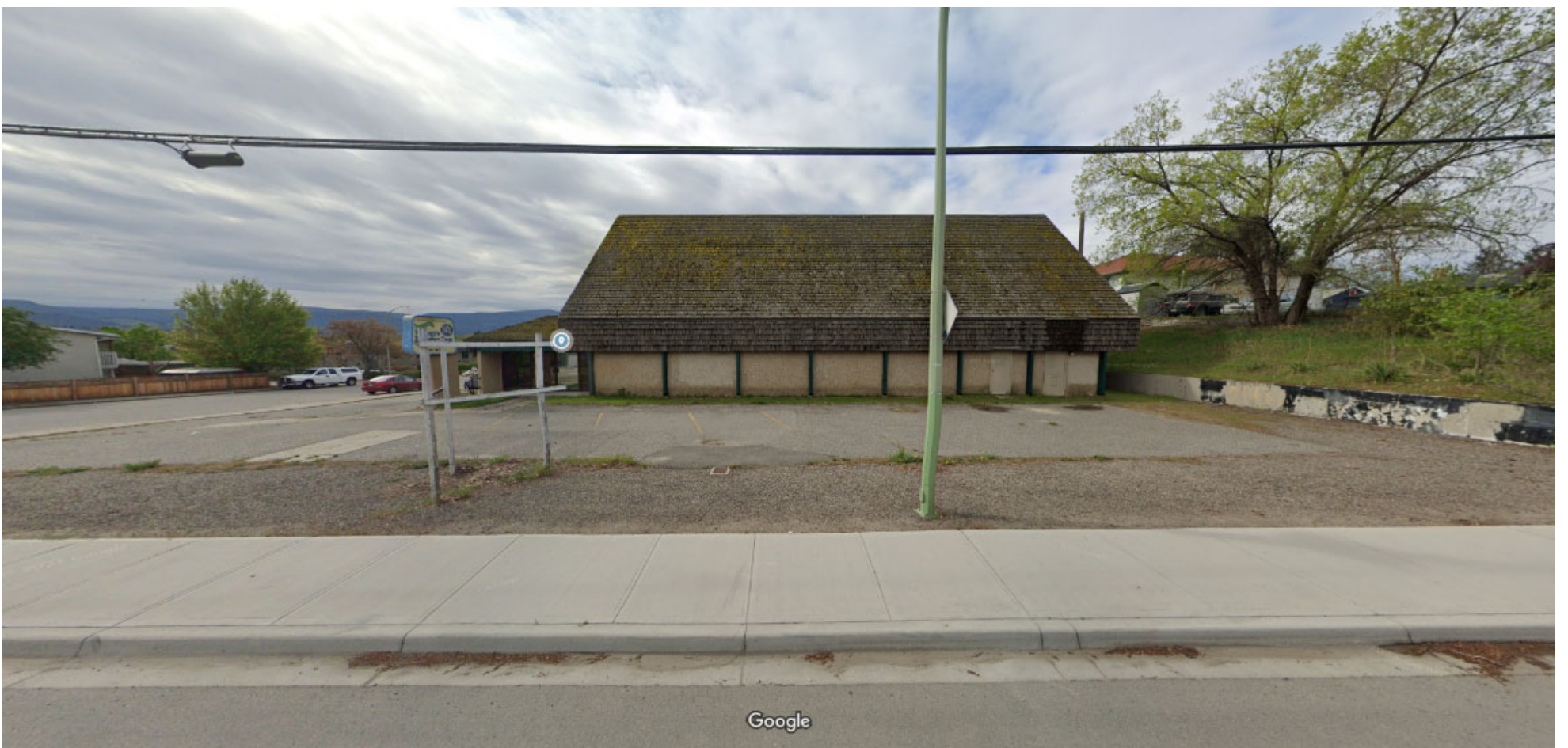
VIEW FROM BERNARD AVENUE - LOOKING SOUTH
