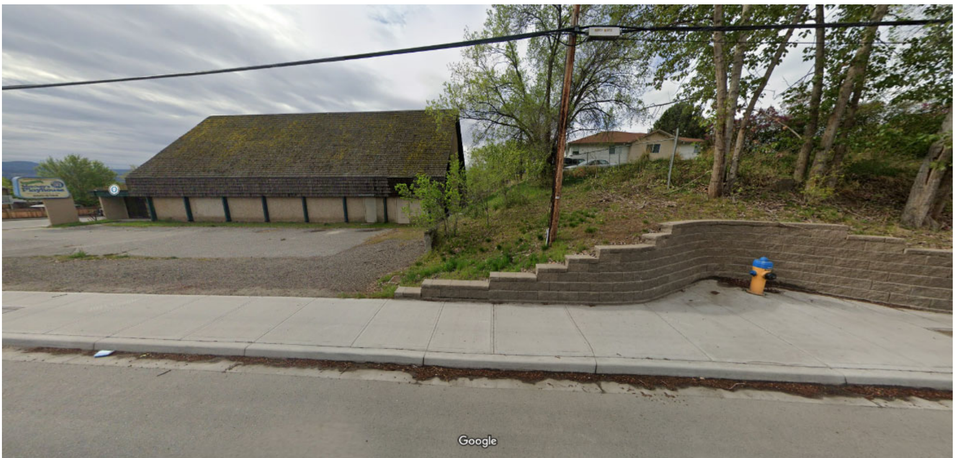
VIEW FROM BERNARD AVENUE - LOOKING SOUTH
