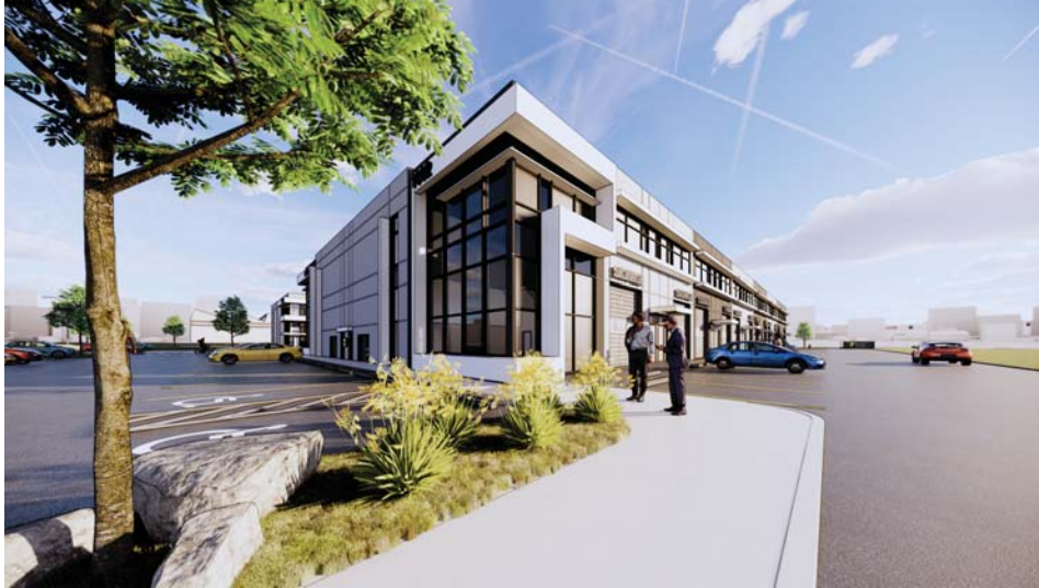
VIEW FROM NORTH ENTRANCE
