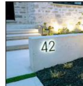
HOUSE NUMBER & CONCRETE WALL
