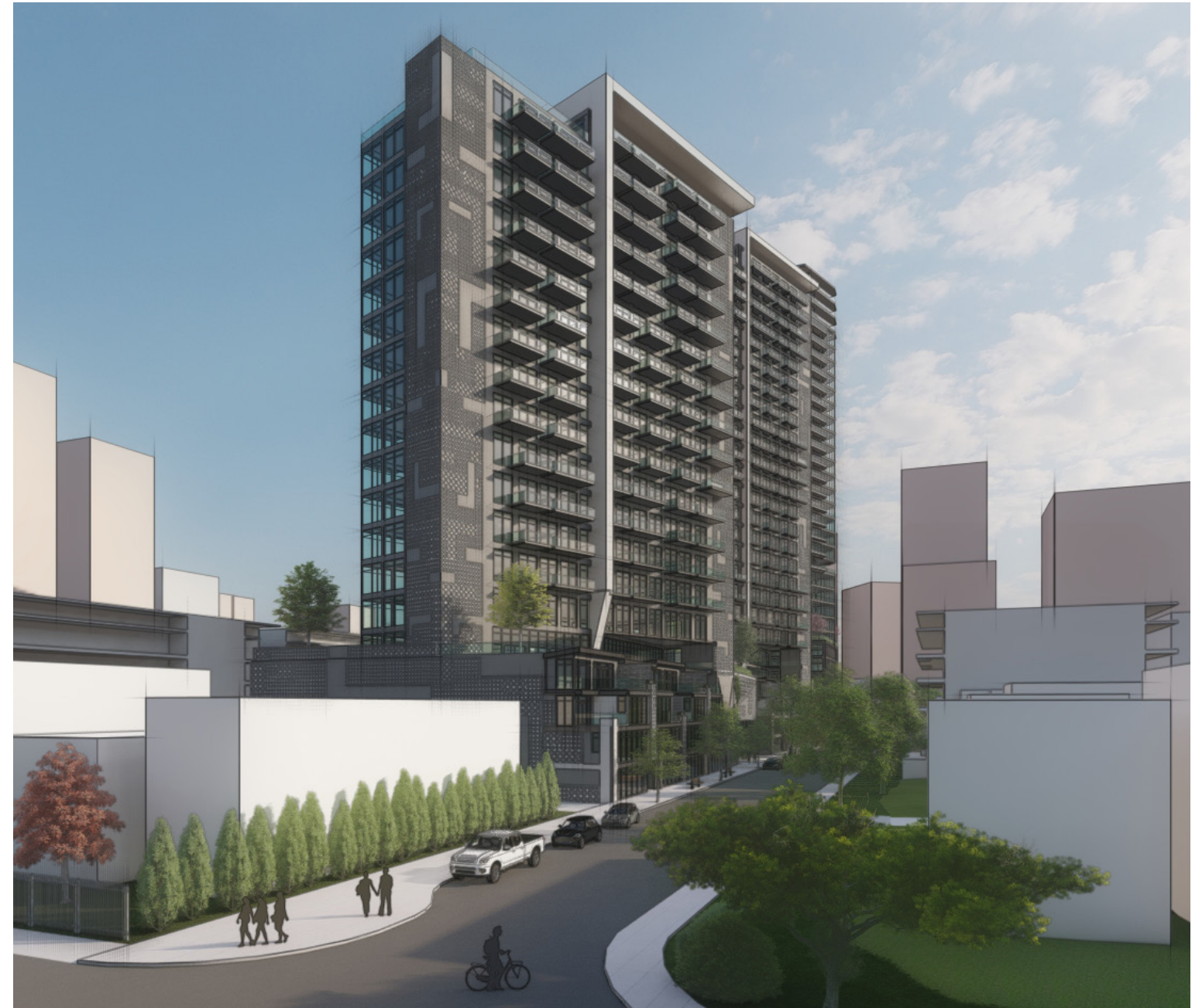
View of proposed rental tower and market townhouses from the intersection of Coronation Avenue and Richter Street.
