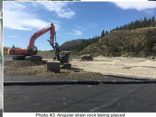
Photo #2: Angular drain rock being placed
