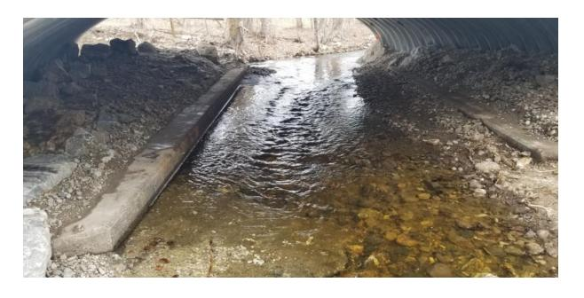
Replacement of the timber bridge circa 1950's along Old Vernon Rd at Mill Creek. The improvements include a new 11.0m x 3.1m arch culvert able to accommodate 17.5 m3/s instantaneous flow which results in raising the road grades 1.2m for a total distance of approx. 250m in length. Budget \$1.5M
