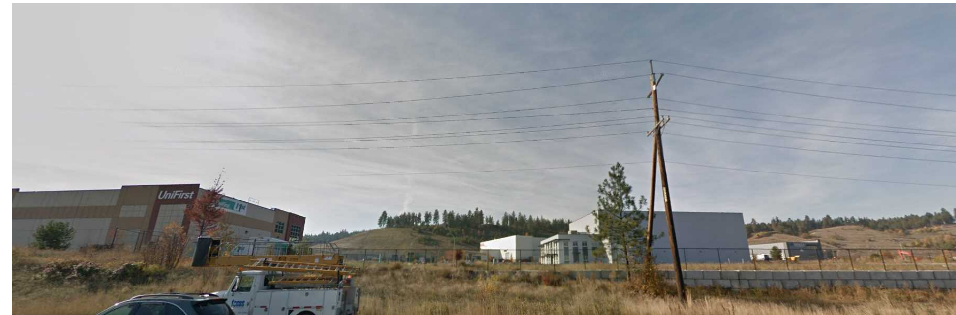
5 VIEW LOOKING WEST FROM HWY. 97 SCALE: NTS
