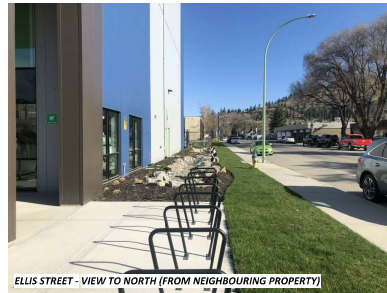
ELLIS STREET - VIEW TO NORTH (FROM NEIGHBOURING PROPERTY)
