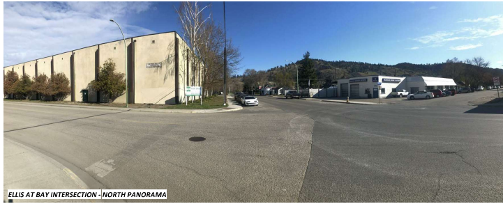
ELLIS AT BAY INTERSECTION -NORTH PANORAMA
