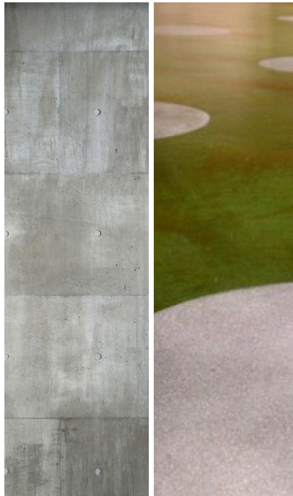
EXTERIOR WALLS STAINED W/ COLOURED CONCRETE SEALER
