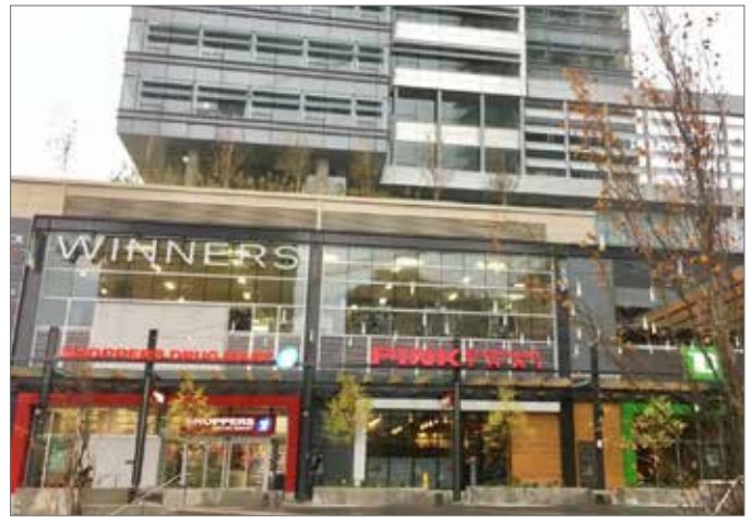
Figure 59: Example of a high rise building with active frontages, high quality materials, and clearly articulated and differentiated podium and tower.
