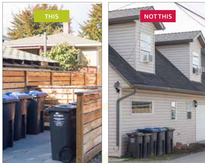
Figure 35: Ensure that site layouts include provision for solid waste pick-up and bin storage that is enclosed or otherwise screened from view (3.3.5. b).
