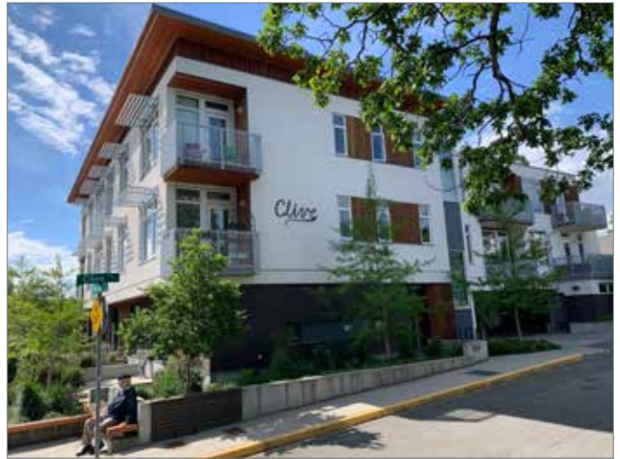
Figure 36: Provide access to parking from the lane or secondary street, and integrate vehicular entrances into the building (4.1.4 a).
