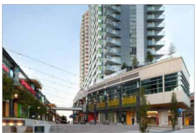
Figure 54: Example of incorporating publicly accessible open space animated by active podium frontages (5.1.5 a-e).
