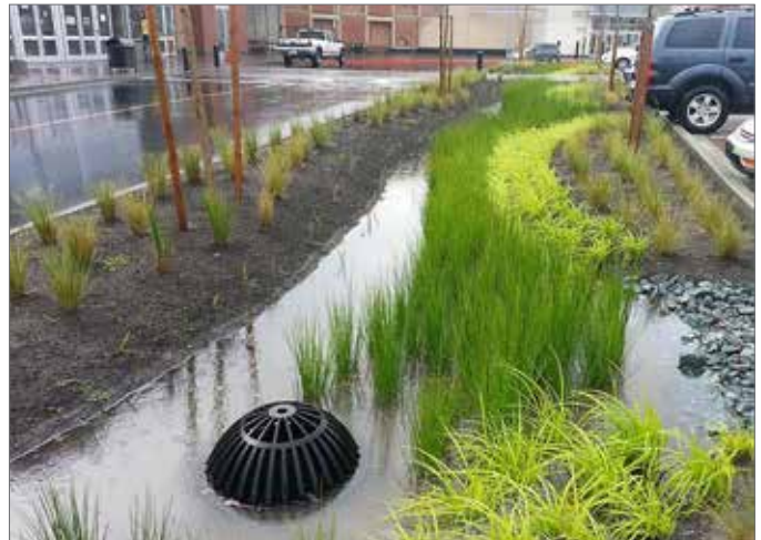
Figure 62: Landscaped areas with rain gardens break up large parking spaces, and provide opportunities for on-site stormwater management (6.1.2 d).
