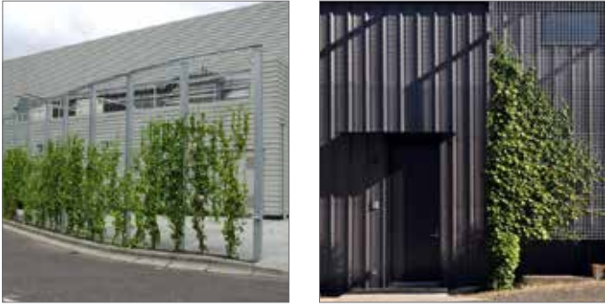
Figure 75: An example of using planting to screen loading and mechanical equipment (left) and enliven facades (right) (6.4.4 a)
