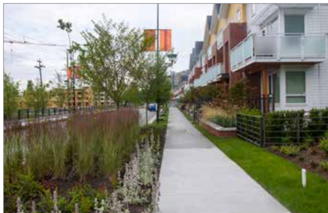
Figure 11: Design sites and landscapes to maintain pre-development flows using strategies such as rain gardens and permeable surfacing (2.1.5 i).
