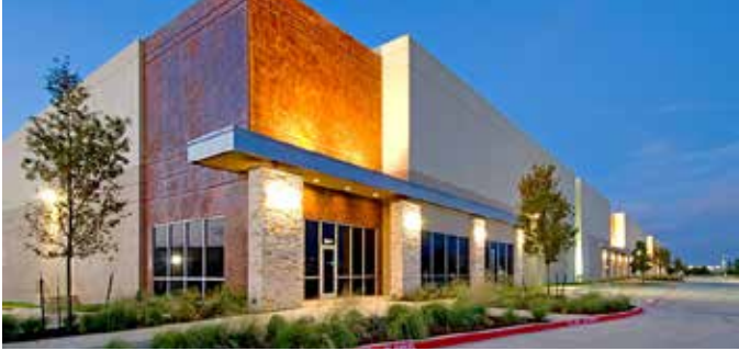
Figure 76: Use of different exterior materials to distinguish between the plant/warehouse component of a building from the office/sales component (6.4.4 b).
