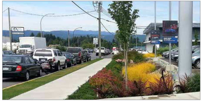
Figure 73: Landscape strip with rain garden adjacent to front visitor parking to provide stormwater management and soften the property edge.
