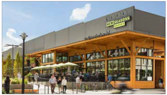
Figure 66: Example of a retail building with a transparent frontage, integrated weather protection and use of natural building materials (6.2.4 b and i).
