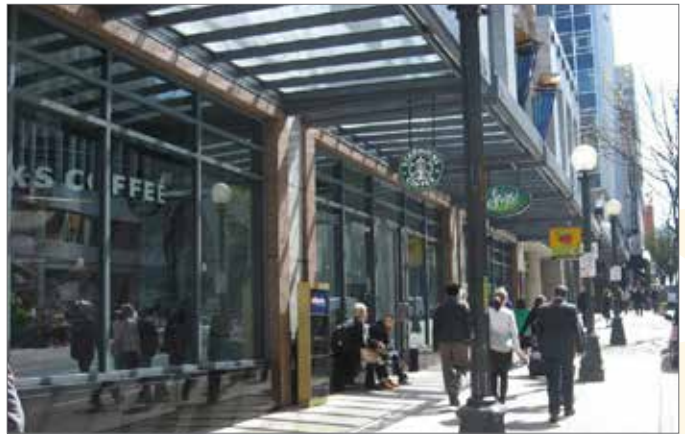
Figure 42: Weather protection and clear signage should be provided along all commercial streets and plazas, and be architecturally-integrated to reflect the pattern of shop fronts and upper storey fenestration/articulation (4.1.6 f-j).
