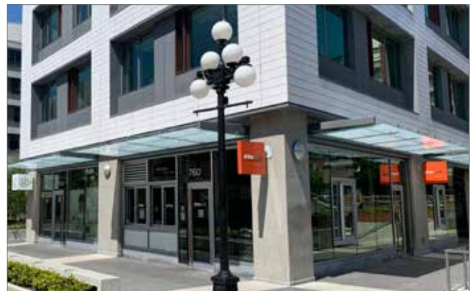
Figure 44: Example of active podium frontage with retail wrapping from primary (left) to secondary (right) frontages (5.1.1 b).
