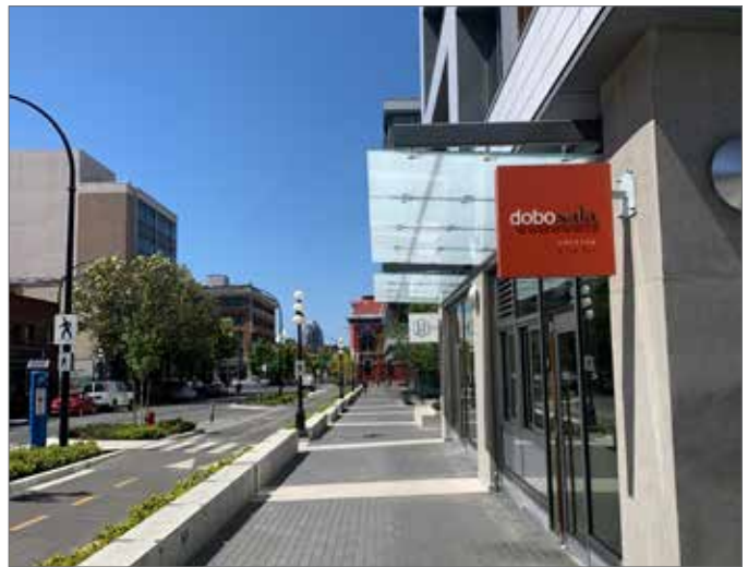
Figure 58: Example of a podium with integrated weather protection and signage at grade (5.1.6. f).
