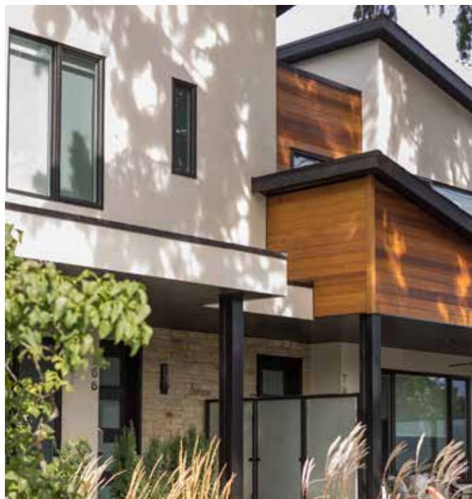
Figure 30: Break down the massing of large buildings through articulation of individual units and avoid symmetry (3.3.2 c, d).
