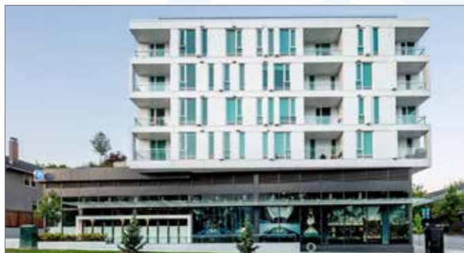
Figure 15: Example of a building with active frontage and low WWR above.
