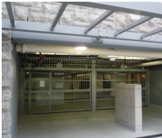
Unobtrusive Parkade Entry
