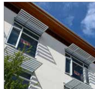
Figure 16: Exterior shading devices can be integrated into a building's southern elevation to block unwanted solar gains and keep indoor temperatures comfortable in warmer months (2.2.1 e).
