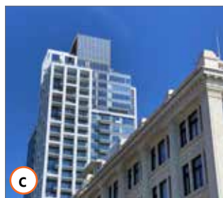
Figure 60: Examples of different approaches to terminating the top of towers: [a] setback on upper floors with architectural feature; [b] architectural lighting; [c] rooftop amenity space with change in materials; [d] screening of mechanical equipment with integrated architectural feature (5.1.6.6 i-j).
