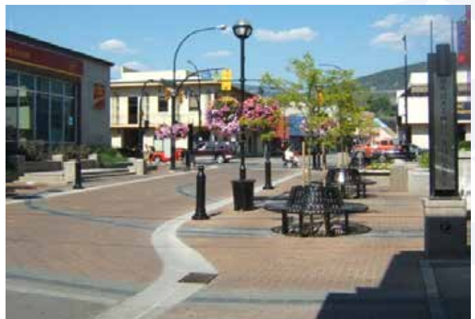
Rolled Curb with Brick Pavers
