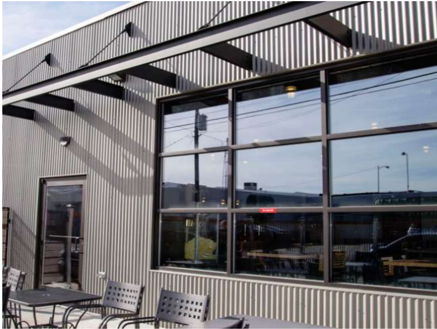
VERTICAL (#3) PROFILED METAL CLADDING - GALVANISED
