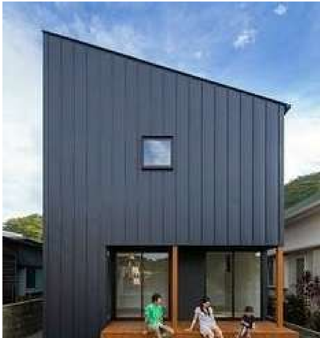
VERTICAL (#3) PROFILED METAL CLADDING - GALVANISED
