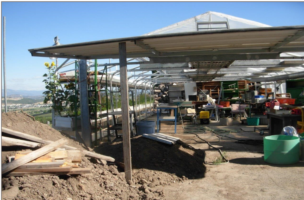
Photo 8: Flat slope above upper wall.
