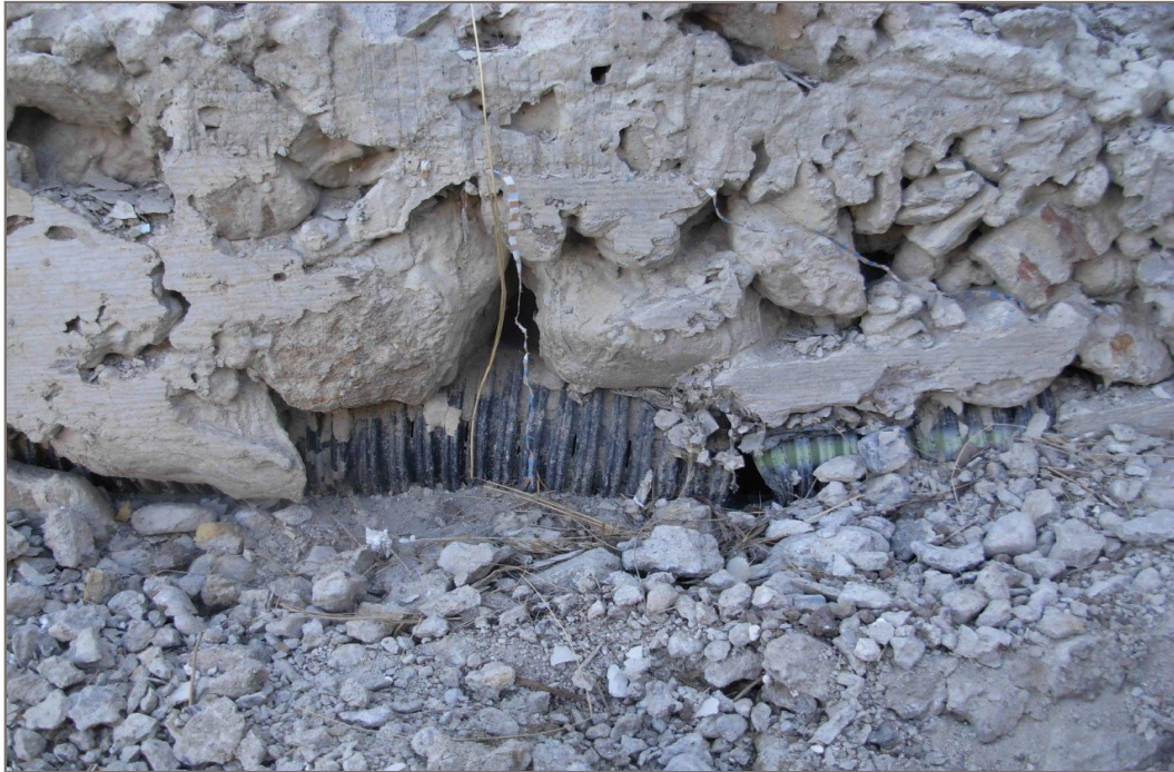
Photo 5: Upper wall south end. Weeping tile below footing wall.
