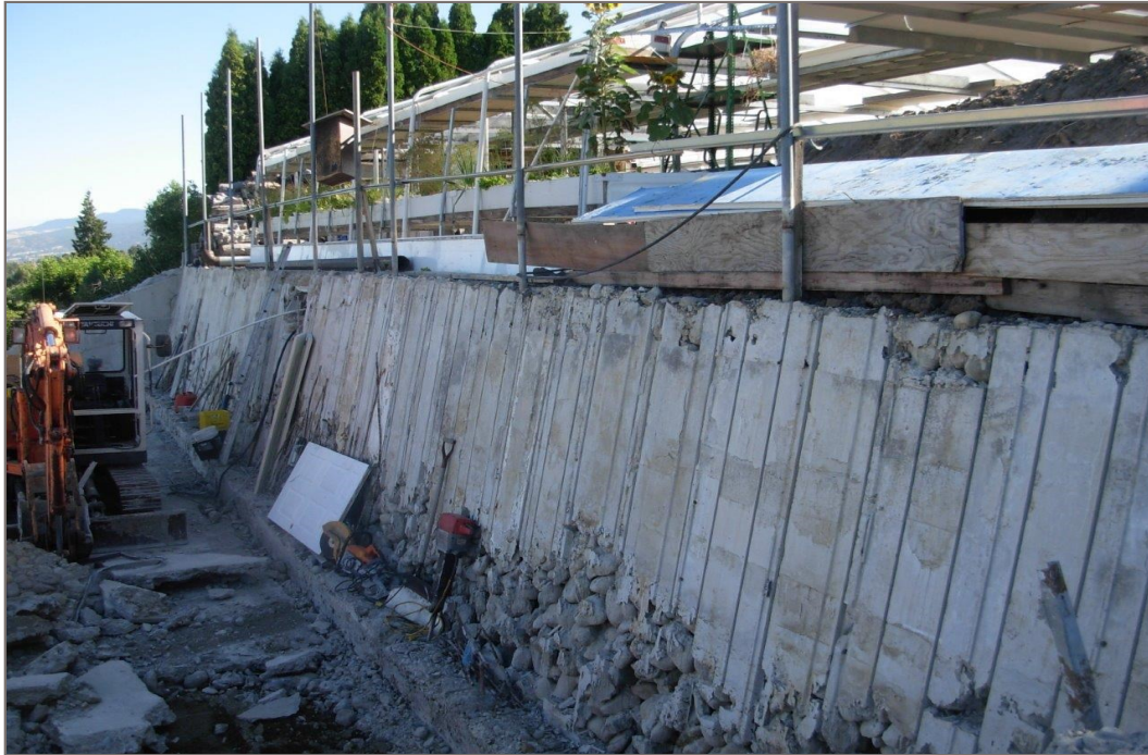
Photo 1: Upper wall view to north.
