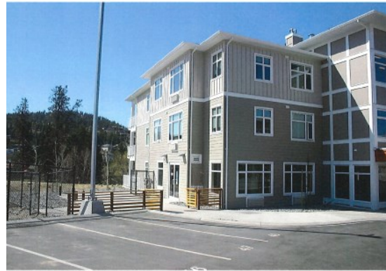
VIEW TO EXISTING ADJACENT EAST APARTMENT BUILDING
