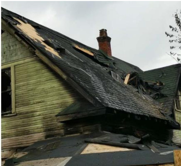
P4: East-south roof
