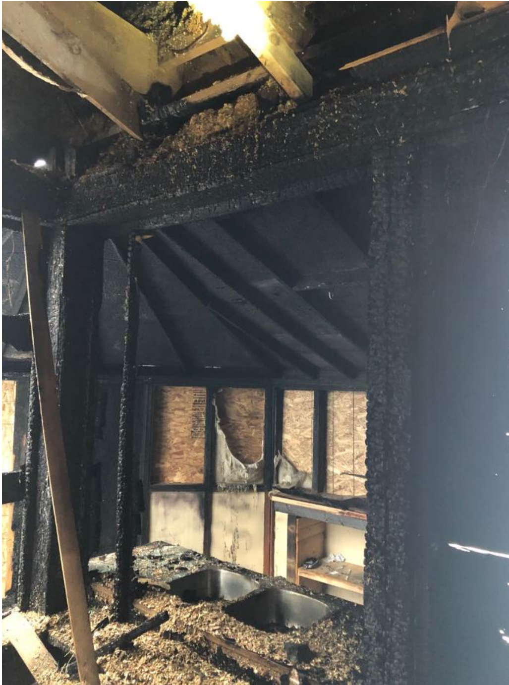
P8: Framing at Kitchen
