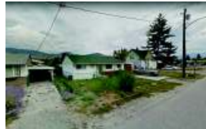
2 SITE PHOTO LOOKING SOUTHEAST
