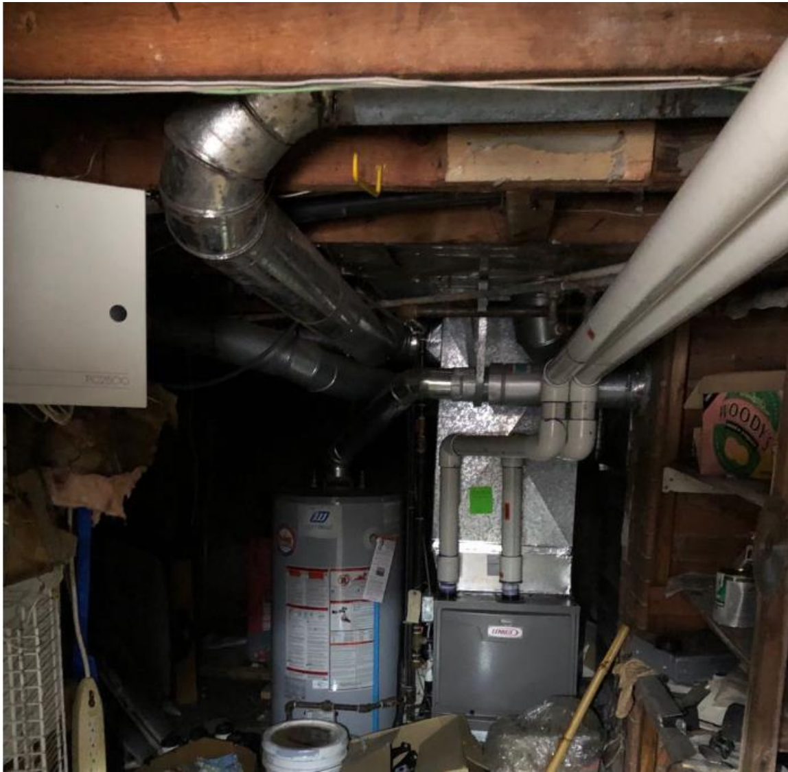
P13: Basement showing main floor framing
