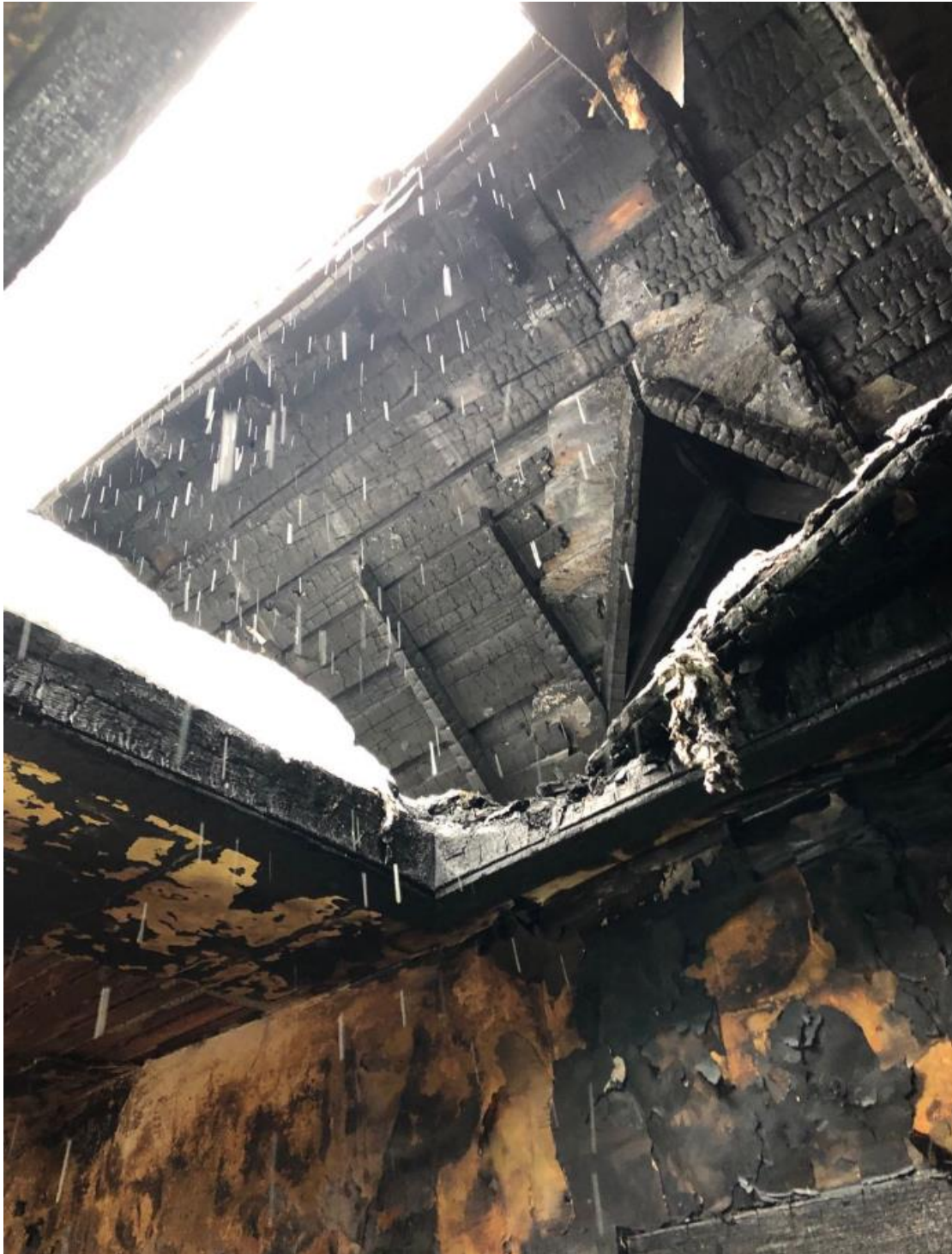
P7: Rafters, ceiling and walls
