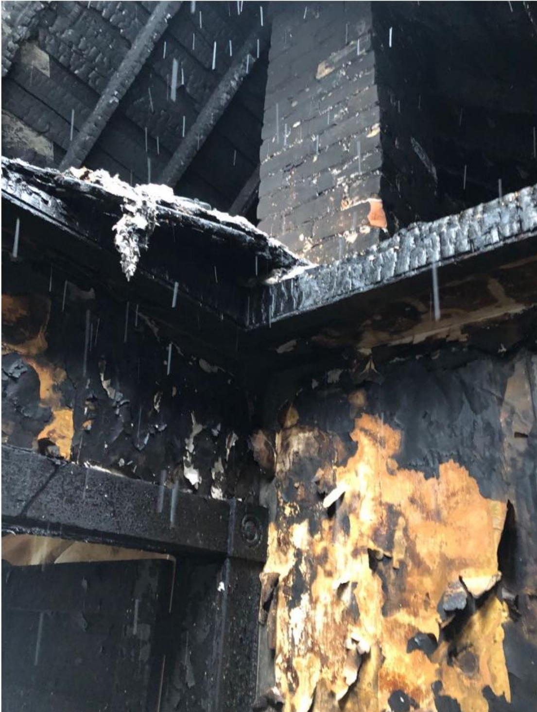
P5: Roof framing around the chimney
