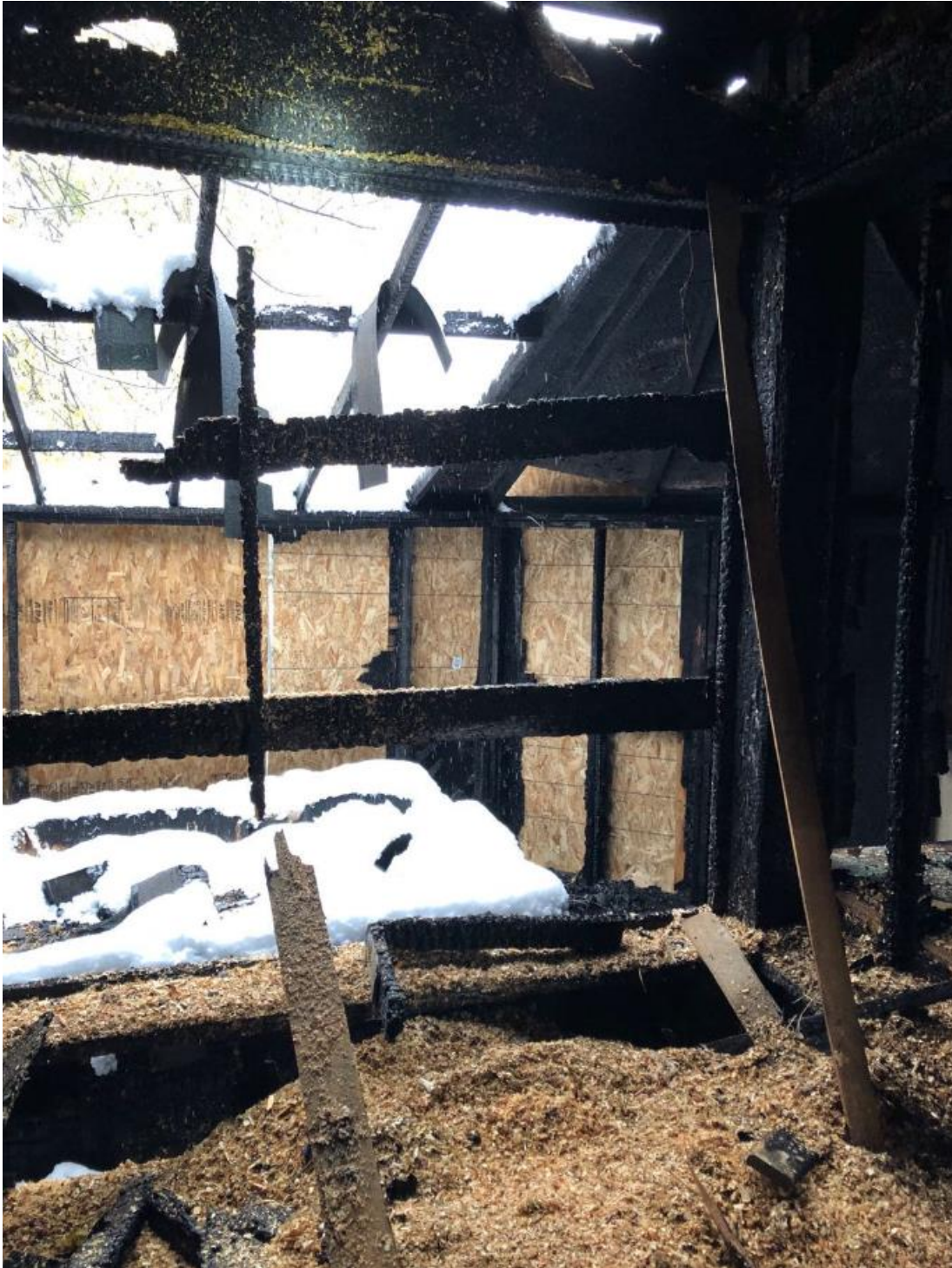
P10: South-east lower roof framing
