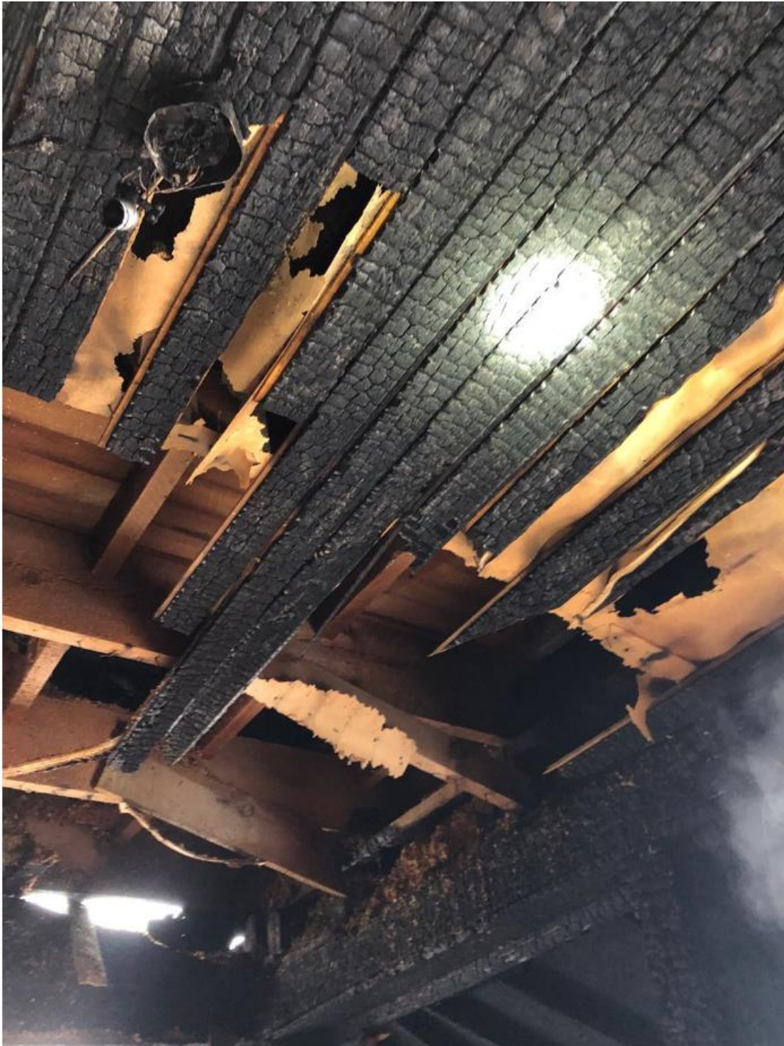
P12: Middle section upper floor
