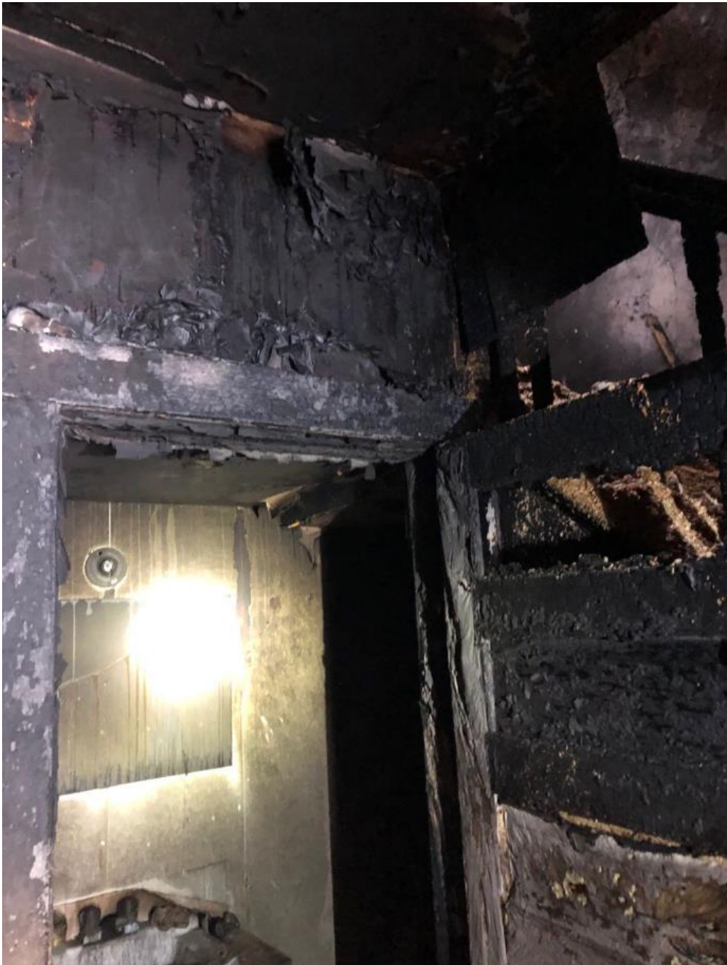
P9: Interior door framing
