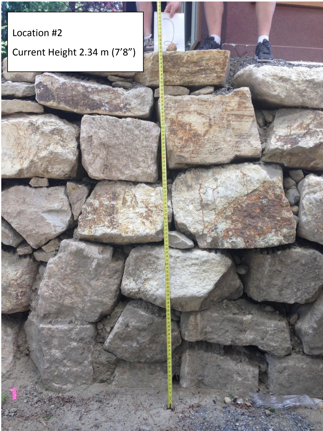
Photo Four: Current retaining wall, at Location #2, as identified on Map One
