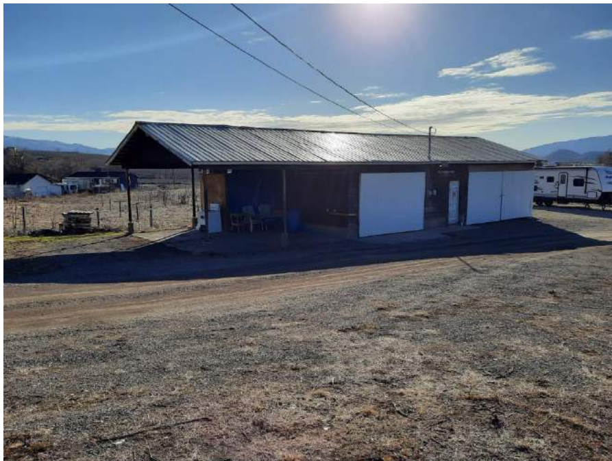
The shed/grapes sales building. Located near the entry to the property.
