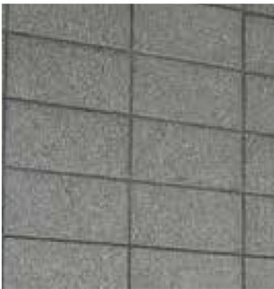
EXISTING STACKED BLOCK WALL
