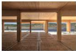
SAMPLE PHOTO CLT - Cross Laminated Timber Construction
