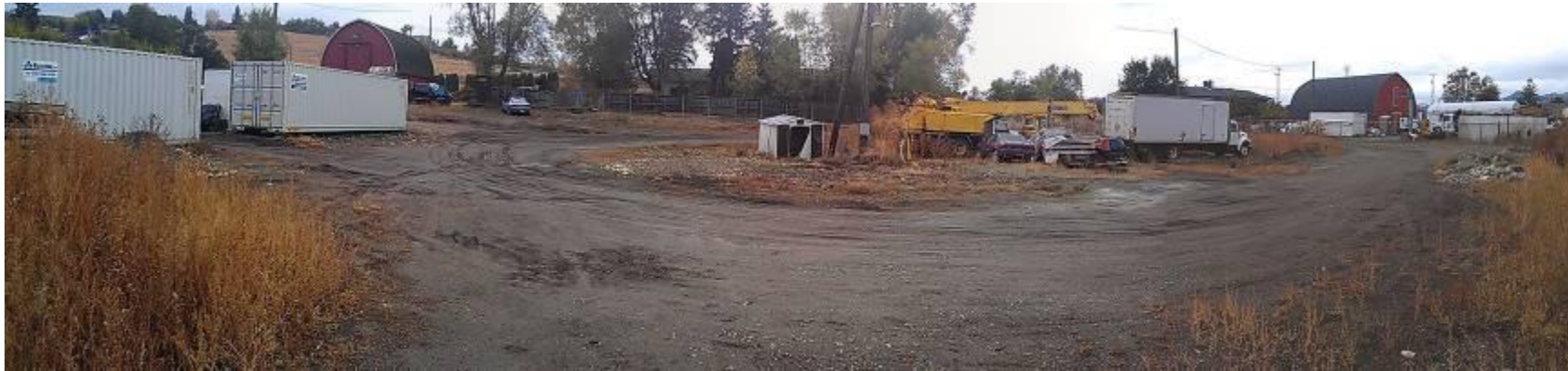
Photo 1: South portion of the site showing remaining footprint of mill work, stored machinery, storage bins and home site in background
