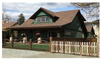
Style: A new house that is in a faux-Craftsmanstyle. Steep side gable roof with a flared eave on the front elevation, front dormer centred on the front elevation with gable roof and a set of three side-by-side multi-pane windows and clad in shingles, horizontal siding on the main body of the house, low horizontal massing, symmetrical, 1 ½ storey, multi-sash horizontal windows, asphalt shingle roof. Parking is accessed from the rear lane. There is a detached garage at the rear of the property.
