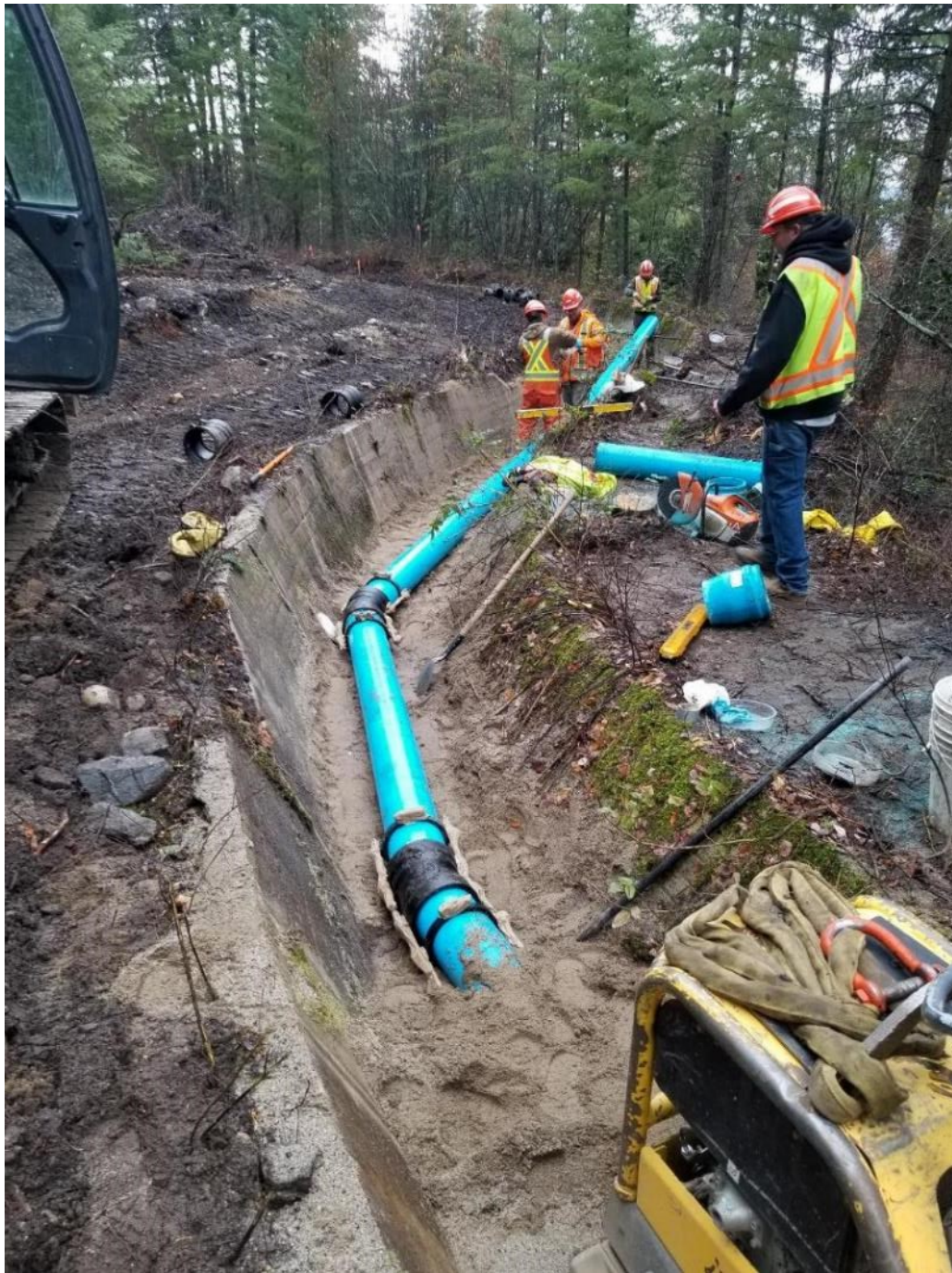
200mm watermain through Myra Bellevue Provincial Park. Alignment making use of abandoned irrigation flume
