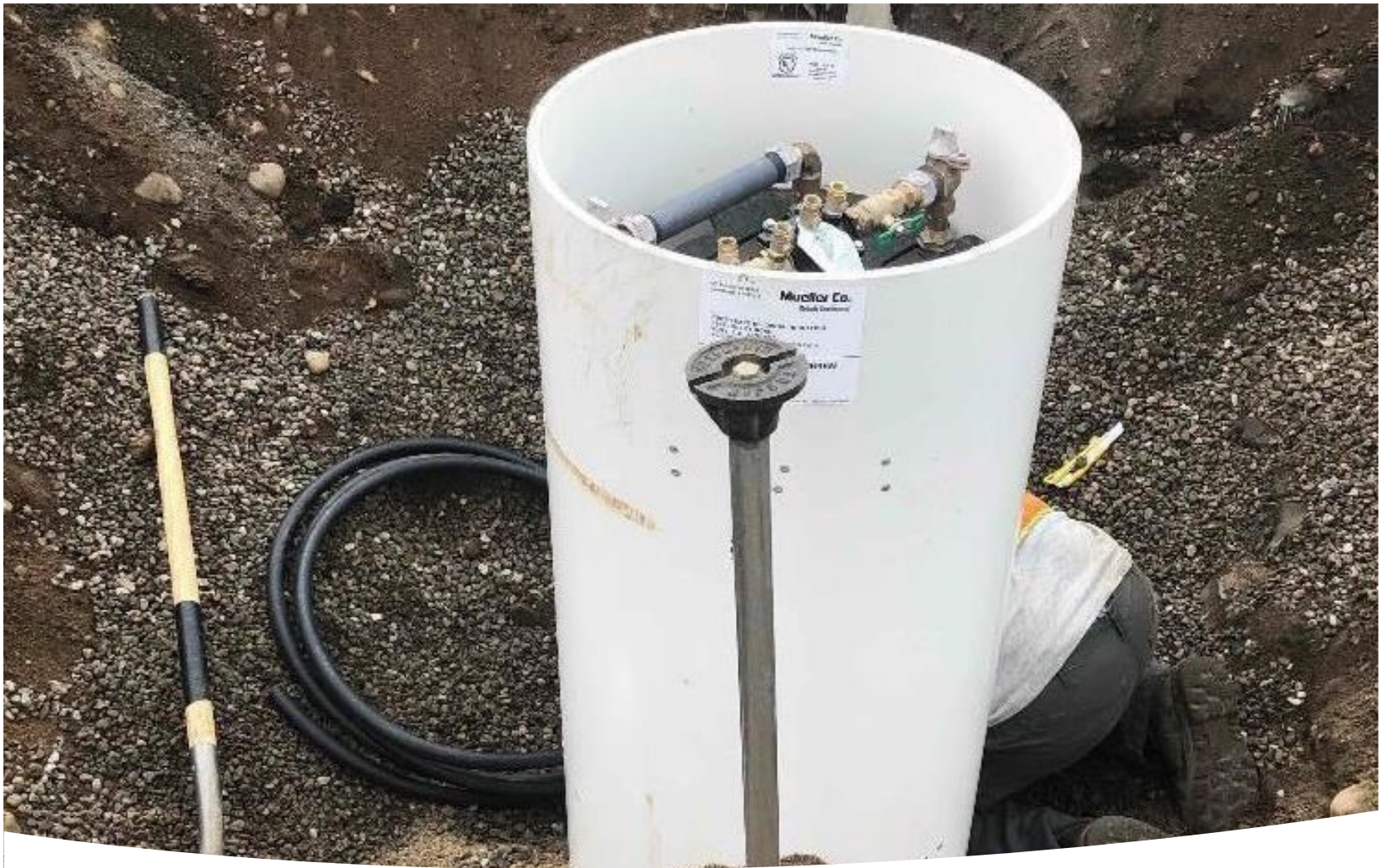
Innovative New Products Mueller Metering Pit with Dual Check Valve Assembly
