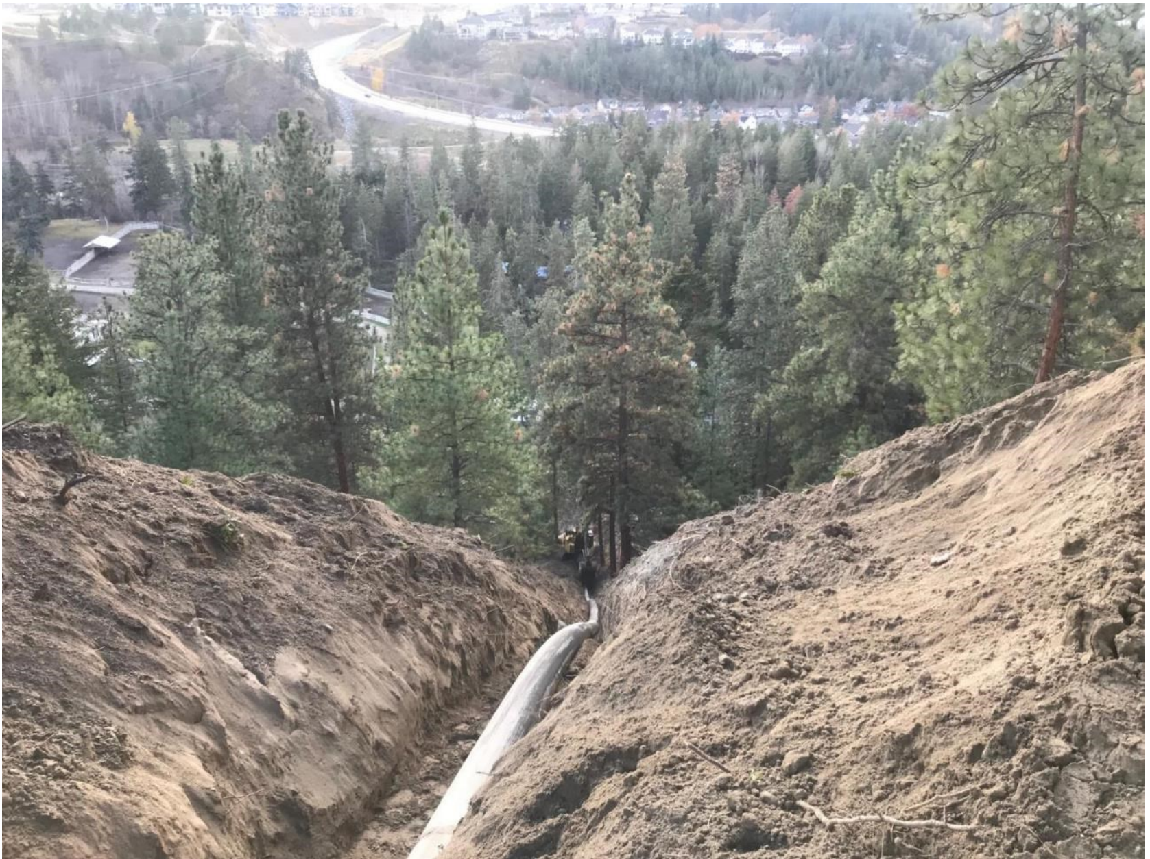
HDPE watermain used in challenging terrain
