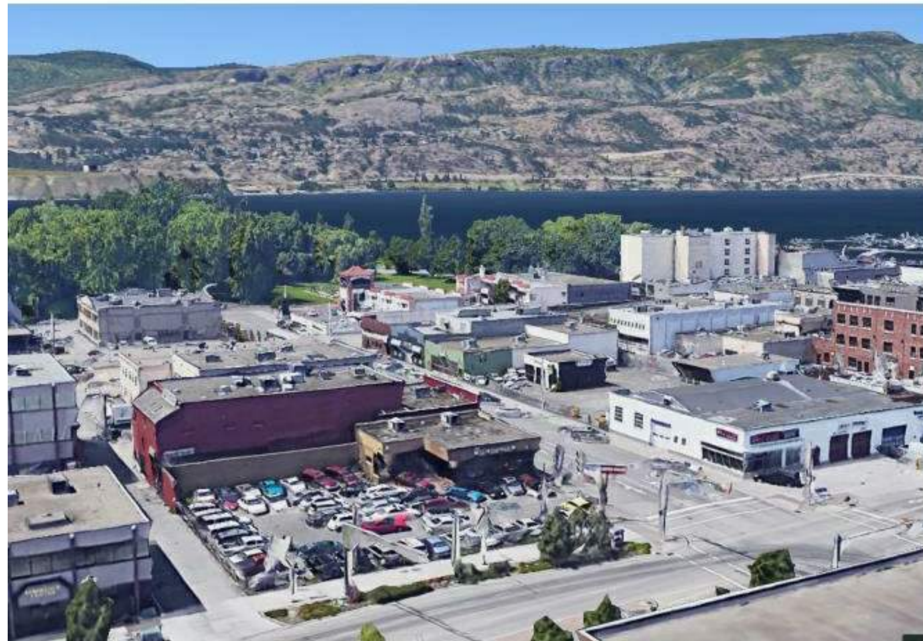
4 - VIEW FROM SOUTH WEST WATER ST / VIEW FROM WATER ST AT SOUTH TOWER
