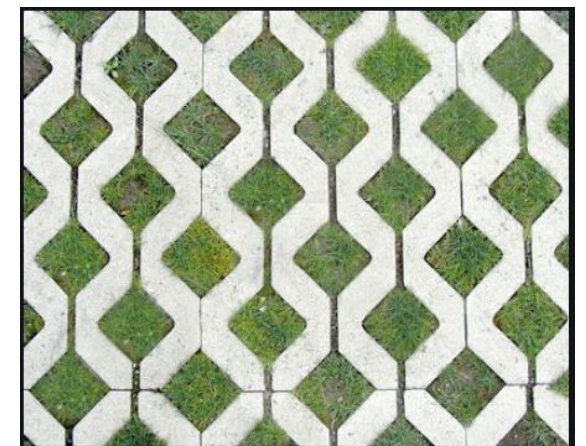
PERMIABLE PAVING
