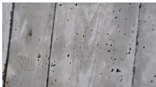
ARCHITECTURALALLY EXPOSED CONCRETE
