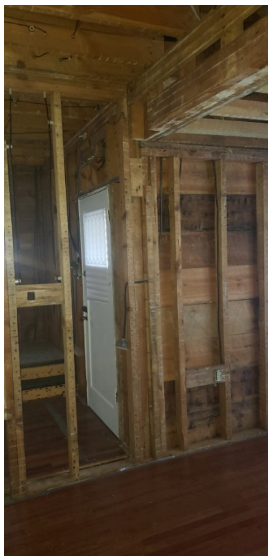
Interior after removal of Lath and Plaster
