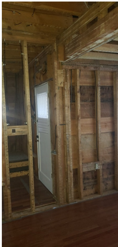
Interior after removal of Lath and Plaster
