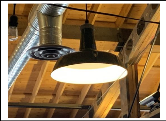
Re-wired light fixture – Laurel Packinghouse
