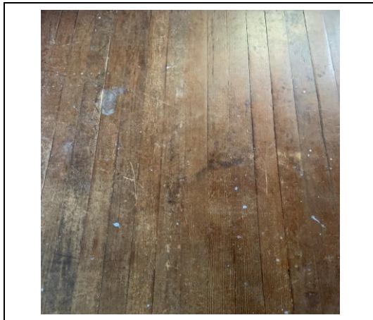
Collett House – fir flooring
