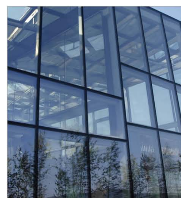
curtain wall glazing
