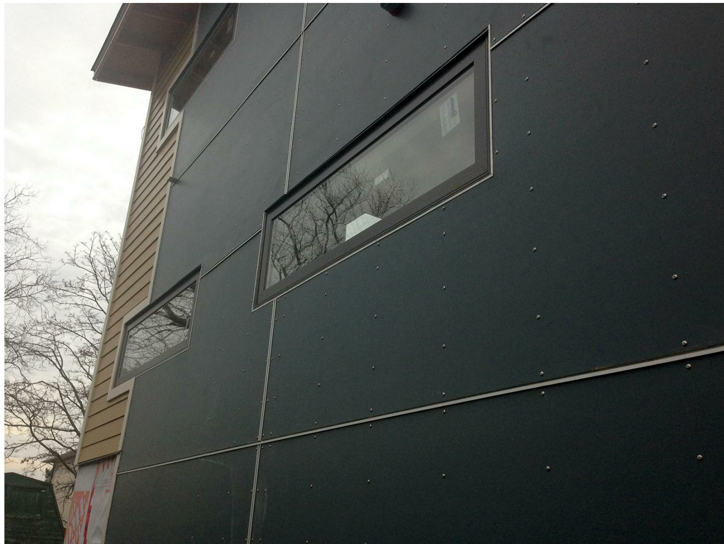
HARDIE PANEL 4'X8' (SMOOTH) COLOR CAVIAR SW6990 W/ EXP. FASTENERS; CORNER TRIMS & BUTT JOINT PAINT TO MATCH (#5)
